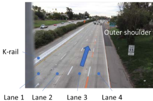
Las Flores bridge, south view, southbound traffic
