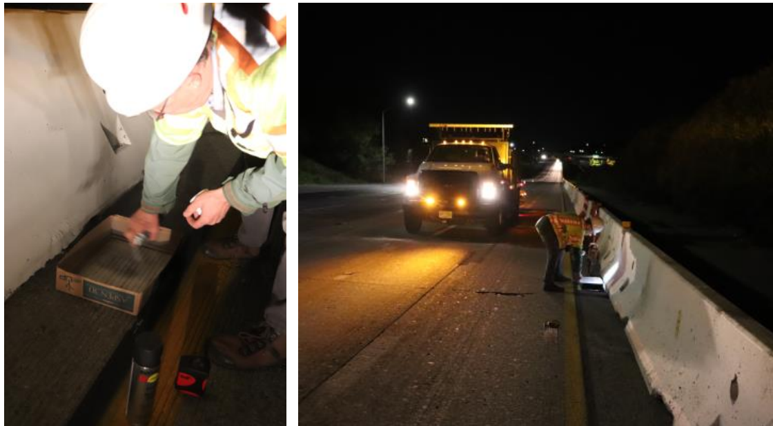
Figure 2.10: Road marking application with spray paint
