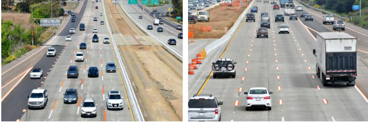
Figure 1.2: Orange preceding white striping in southbound (SB) direction (left); orange along both sides of white striping in northbound (NB) direction (right) (photos: courtesy of Caltrans)
