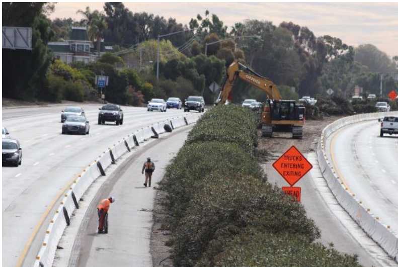
Figure 1.1: Workers in a work zone in the I-5 NCC project
