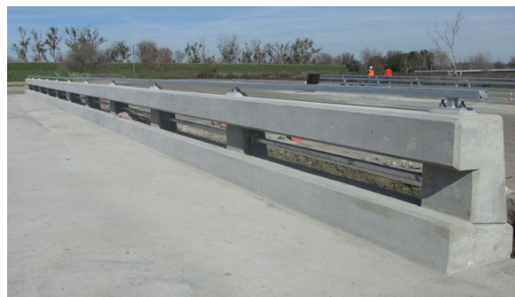
Image 2: Completed Type 85 Bridge Rail at the Caltrans Dynamic Test Facility
