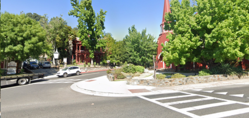
Post-construction with curb bulbs out and accessible ramps
