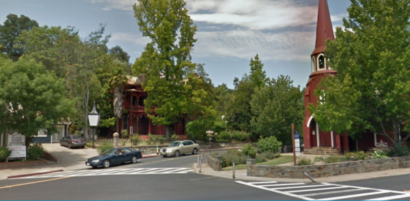
Pre-construction without curb bulbs out and accessible ramps
