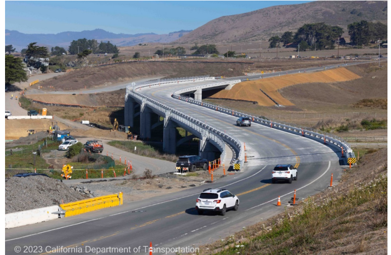
© 2023 California Department of Transportation
