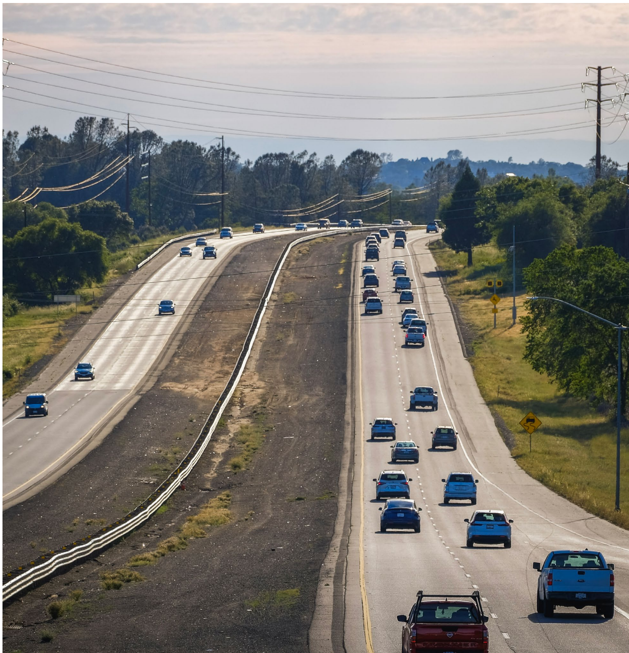
Travel on US 50 near Shingle Springs illustrates the corridor's importance for commuter, recreational, and commercial travel.
