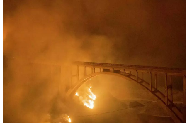
Figure 35 The Colorado Fire burns along Rocky Creek Bridge on State Route 1, District 5. Source: The Associated Press (2022).
