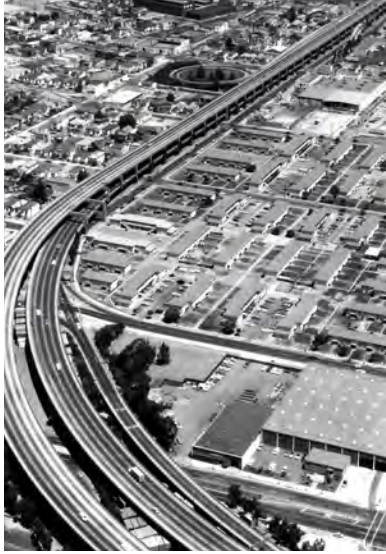
Photo 1: Cypress Street Viaduct in Oakland, CA.
