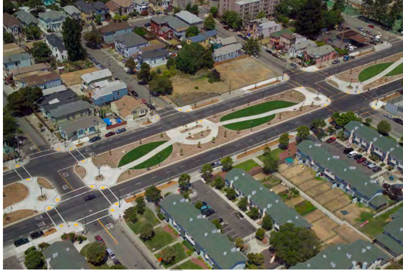
Photo 2: The new Mandela Parkway in Oakland, CA following conversion from the Cypress Street Viaduct.
