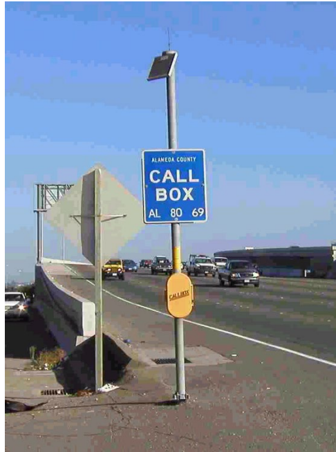
Figure E-8 Site Type H or K – Installed on a K-Rail or Concrete Barrier
