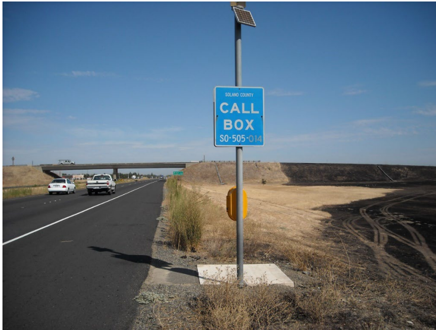
Figure E-2 Site Type B – Installed in a Cut Slope (See Chapter 115, Section 5, Topic 5)
