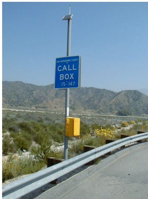
Figure E-6 Site Type F – Installed Behind a Guard Rail
