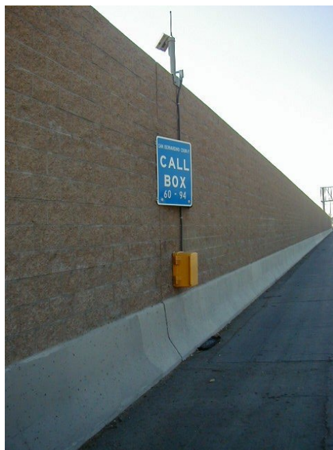
Figure E-4 Site Type D – Mounted on a Soundwall
