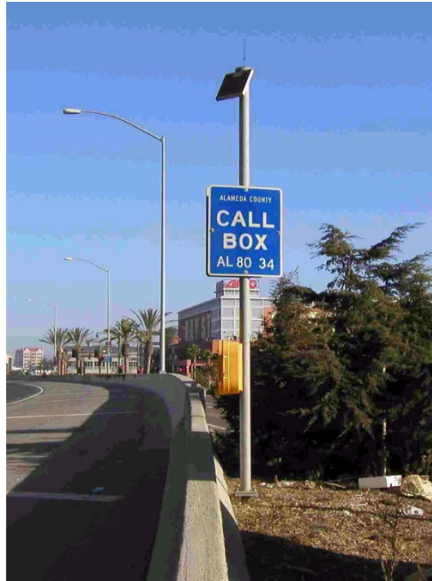
Figure E-6 Site Type F – Installed Behind a Guard Rail
