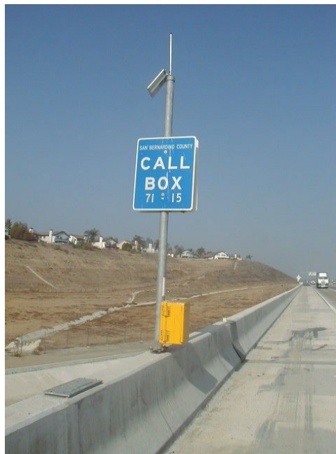
Figure E-8 Site Type H or K – Installed on a K-Rail or Concrete Barrier
