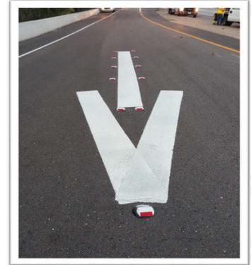
In addition, all ramps that had a Type V Arrow had the arrows modified with the addition of (Clear/Red) or (Blank/Red) Reflective Markings on the Type V ramp pavement arrows.
