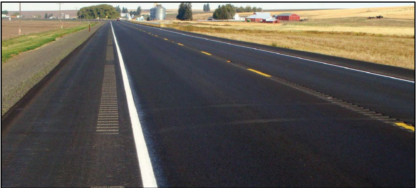
Figure 1: Typical shoulder and centerline rumble strips where bicycles are permitted.
