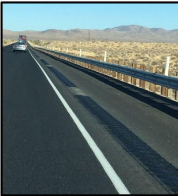
Figure 6: Photo of shoulder rumble strip gaps for bicycle to traverse rumble strip
