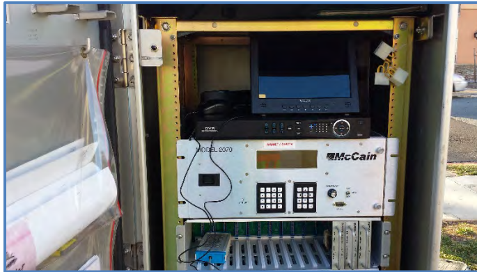
Figure 3 – DVR and monitor placed in signal controller cabinet at Location 4.
