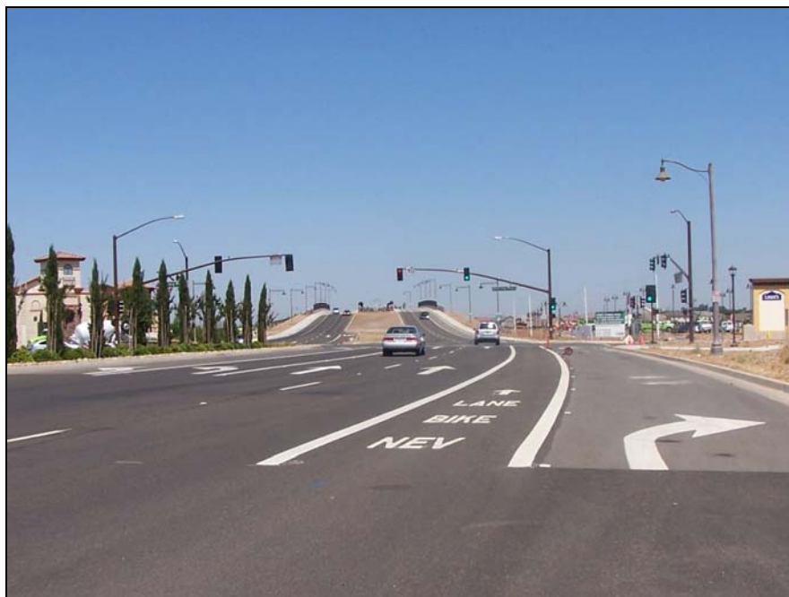
Figure 3. Combination NEV/Bike Lane Pavement Marking and Striping
