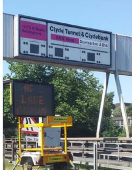
Temporary patching of overhead gantry for GRN wayfinding signage (Glasgow 2014)
