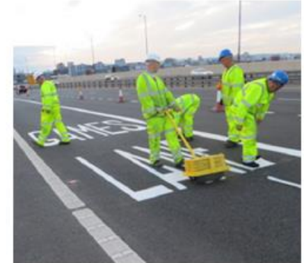
Temporary striping / road marking
