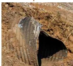
Sinkholes, which are usually caused by "voids" created in the compacted material that surrounds a failed culvert under or around traveled roads, can disrupt the movement of people and goods.
