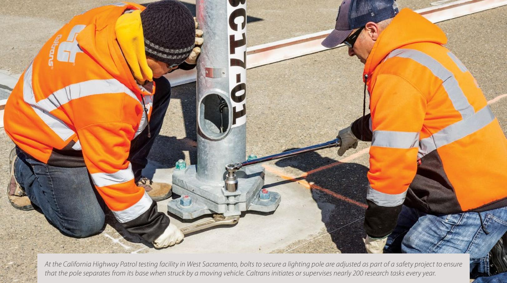
*At the California Highway Patrol testing facility in West Sacramento, bolts to secure a lighting pole are adjusted as part of a safety project to ensure that the pole separates from its base when struck by a moving vehicle. Caltrans initiates or supervises nearly 200 research tasks every year.*
