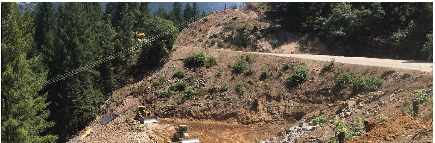
Construction crews fortified this embankment along SR 36 on the east end of the project. The contractor used rock from the work site for slope protection and drainage basins, eliminating the need to haul in material from other places, saving time, money and reducing air pollution.
