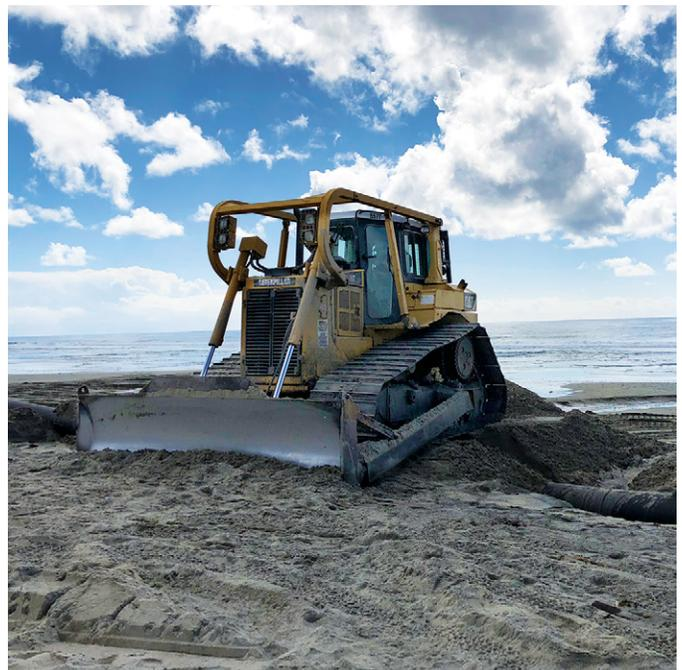
*A bulldozer moves recently pumped sand onto Cardiff State Beach as part of a lagoon restoration project in the San Diego area.*
