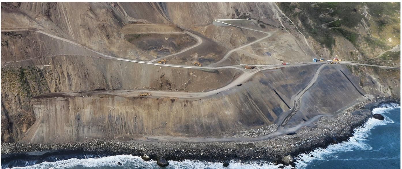
Construction crews create a new roadway base for the middle and north sections of the Mud Creek project. Access roads have been constructed for future maintenance of the site. A rock barricade, called a revetment, was built along the shoreline to keep the tide from eroding the embankments.
