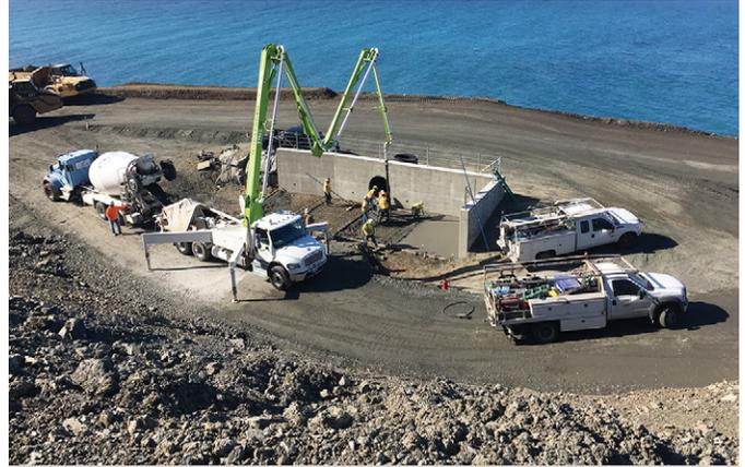
Crews pour a concrete drainage pad under the five-foot-plus diameter pipe that will drain excess water from the Mud Creek area.
