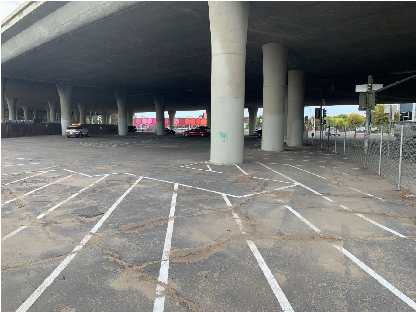
At the northeastern corner of the FLA looking west.
