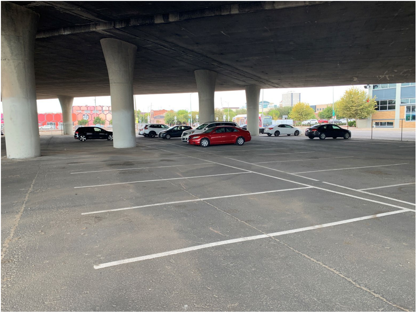
At the eastern corner of the FLA looking northwest.
