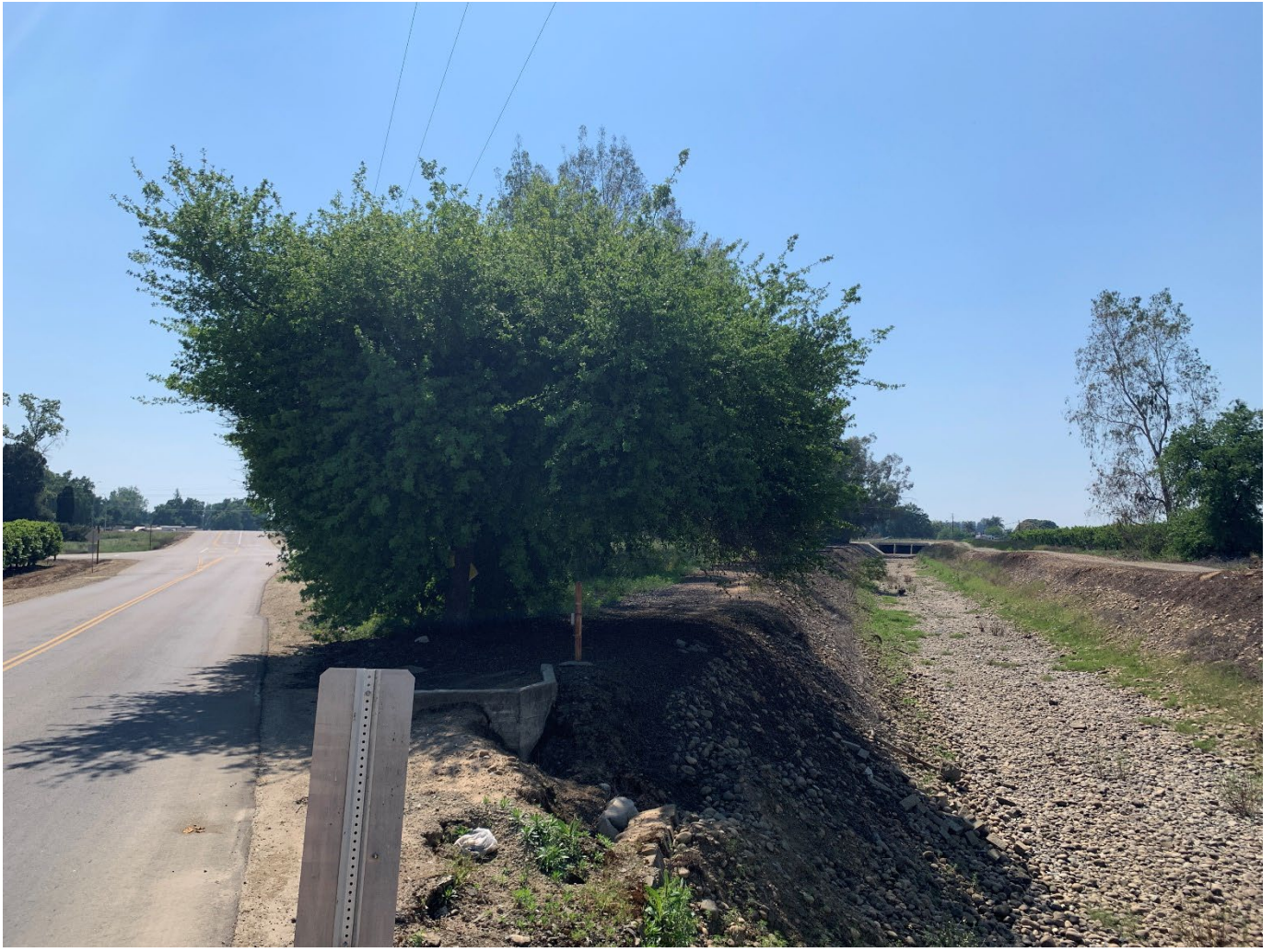
On N Oliver Ave looking southwest at the parcel.
