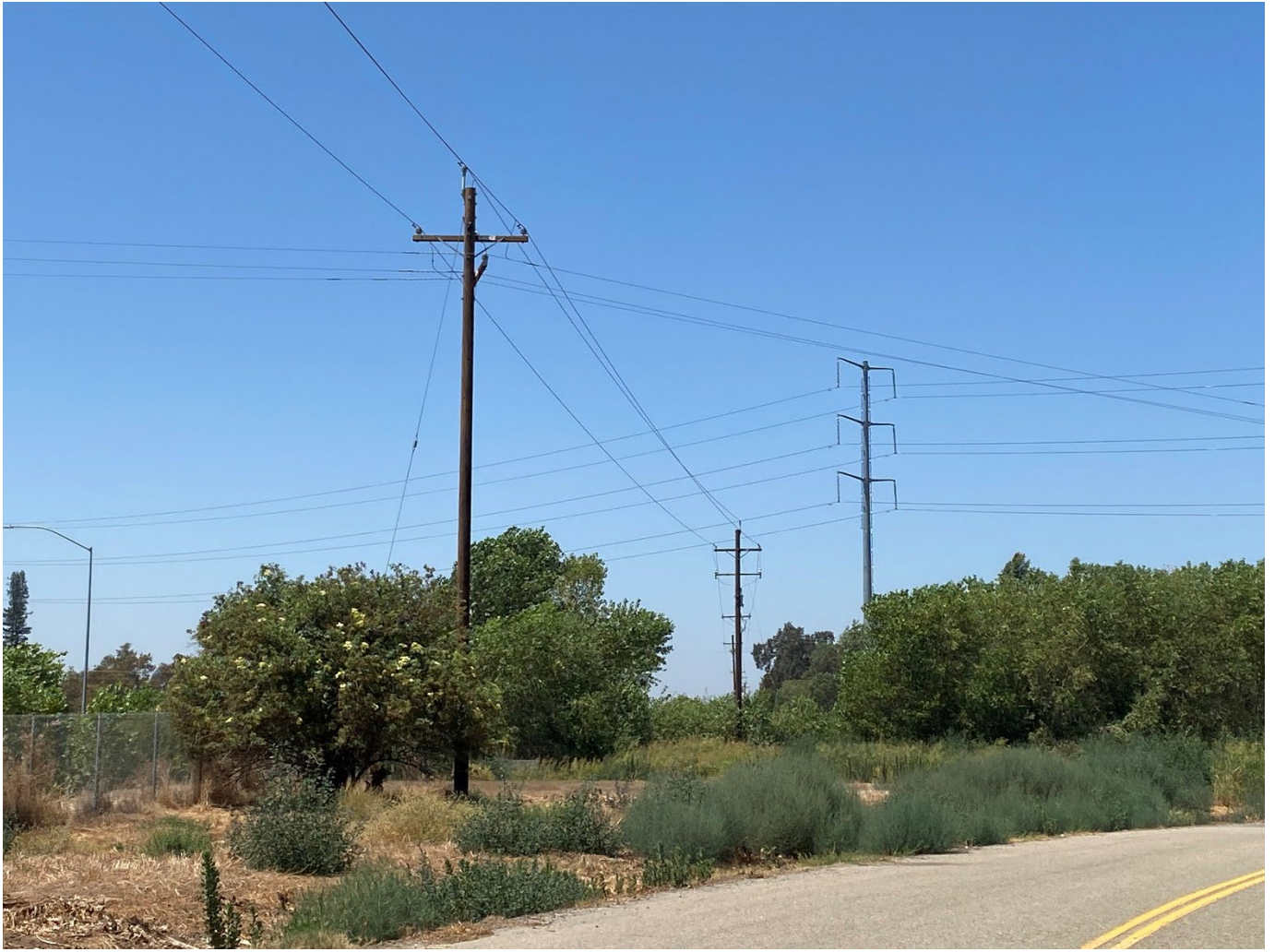
DD 84600-01-01 – Looking west at the parcel.
