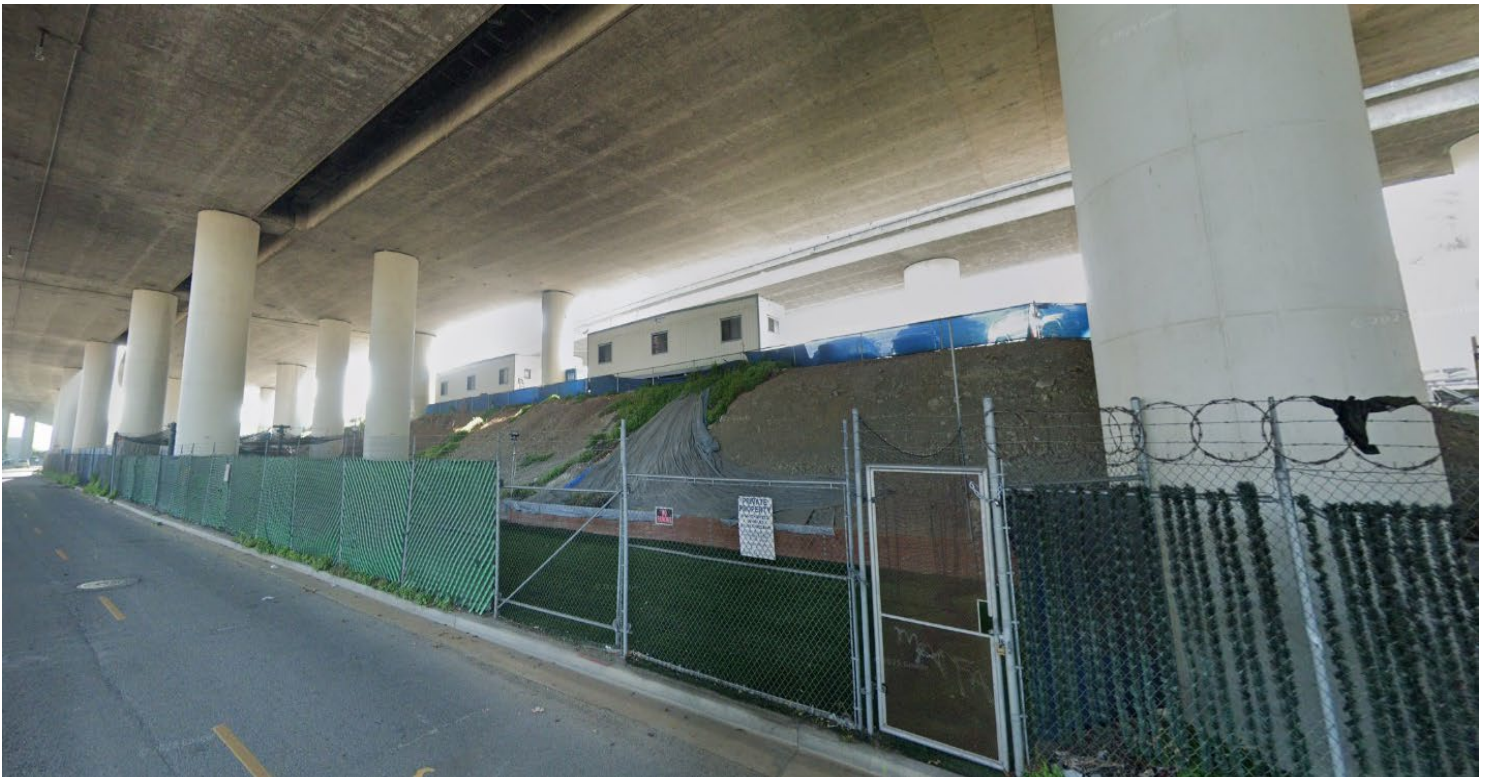
Looking southwest from Iowa Street
