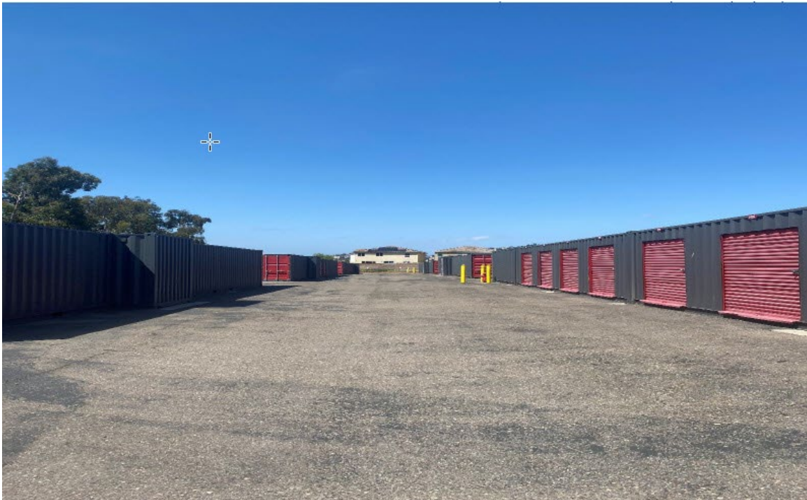
Photo of leased area facing west. Storage units are outfitted cargo containers and considered personal property of tenant
