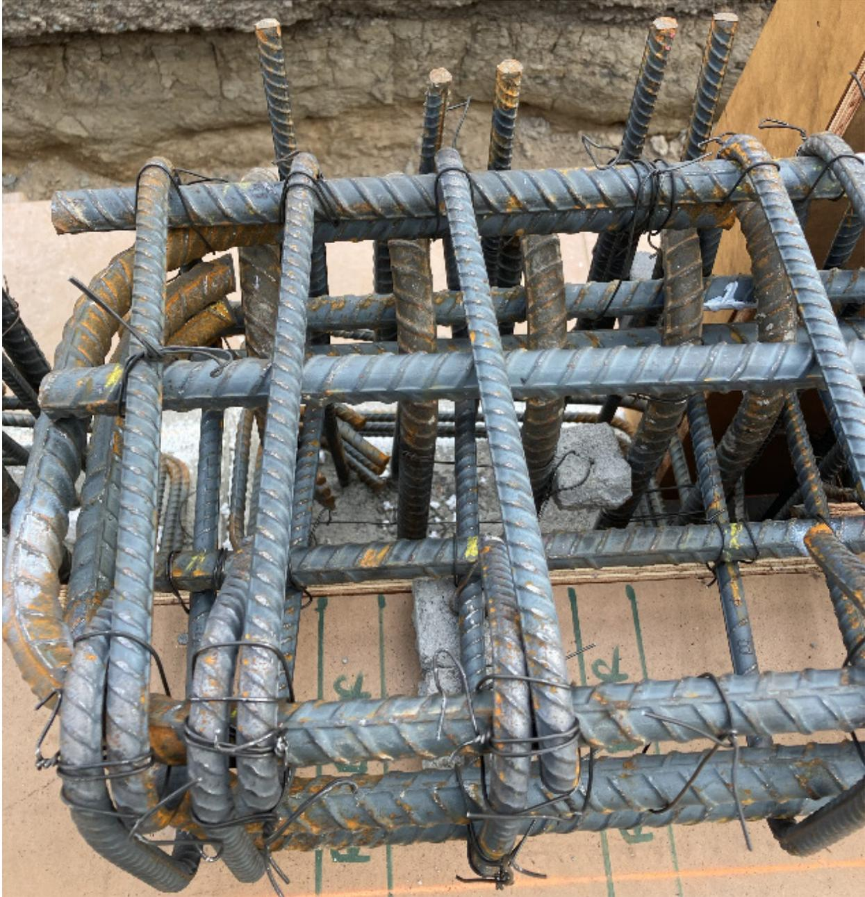
**Figure 2-43 Resolved Conflict and Completion of Installation of Beam Reinforcement at Post 4**
