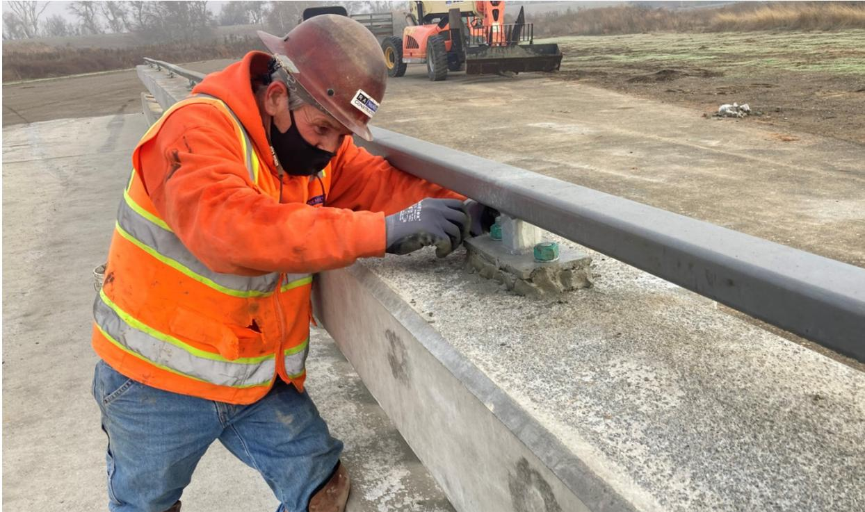
**Figure 2-50 Installation of Tubular Bicycle Railing and Mortar Pad at Supports**
