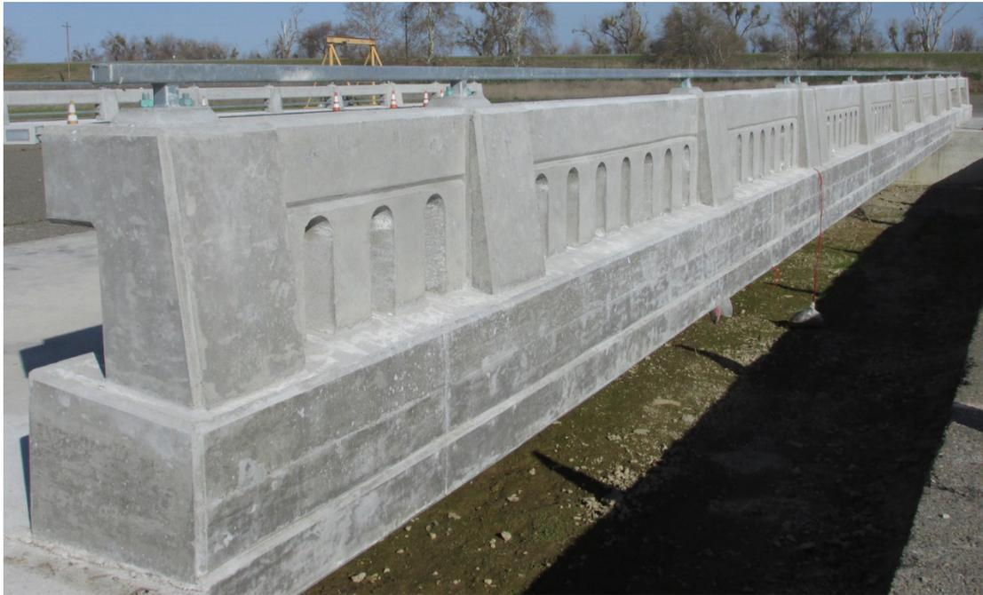
**Figure 1-2 Concrete Barrier Type 86H (Non-Traffic Face)**
