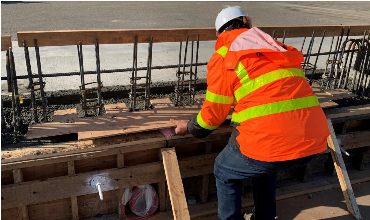
Figure 2-33 Verification of the Placement of the Baluster Rail Reinforcement Using Plywood Template
