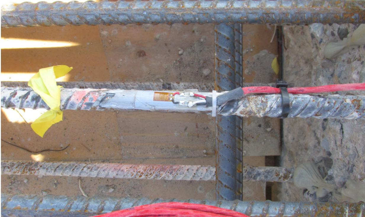
Figure 2-21 Installation of Uniaxial Strain Gauges and Cable Prior to Deck Pour
