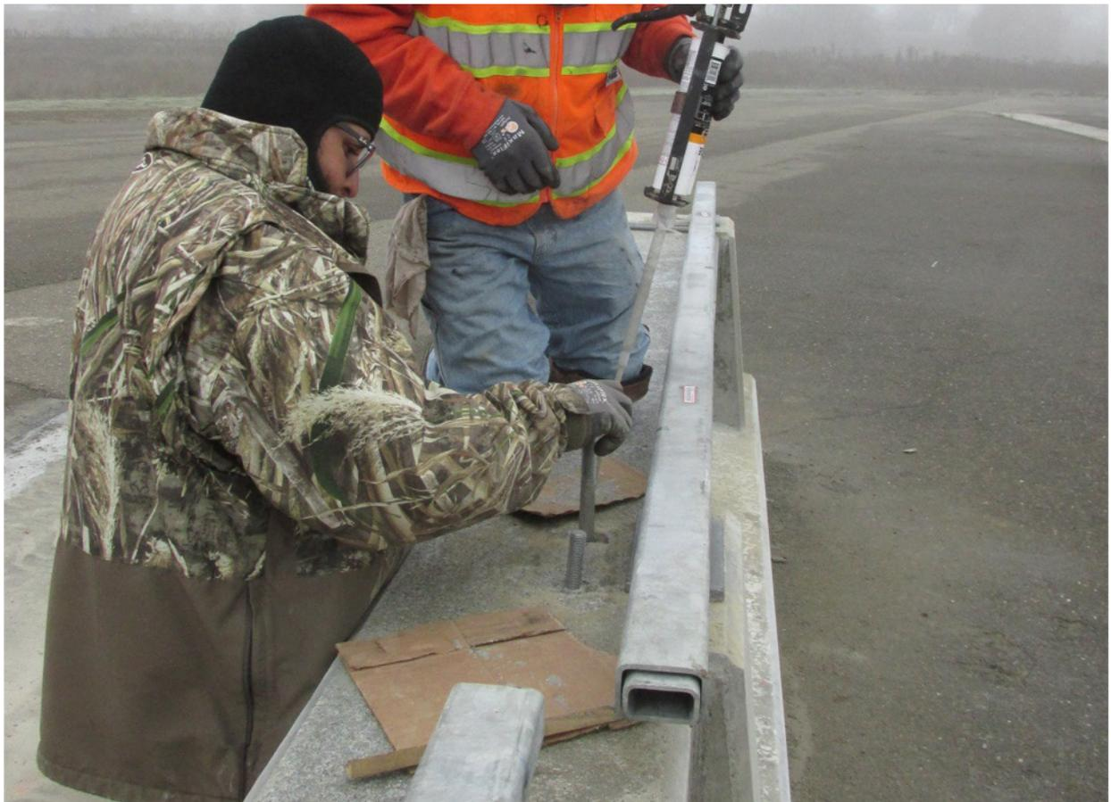
Figure 2-49 Drilling and Bonding of the Threaded Rods for Tubular Bicycle Railing
