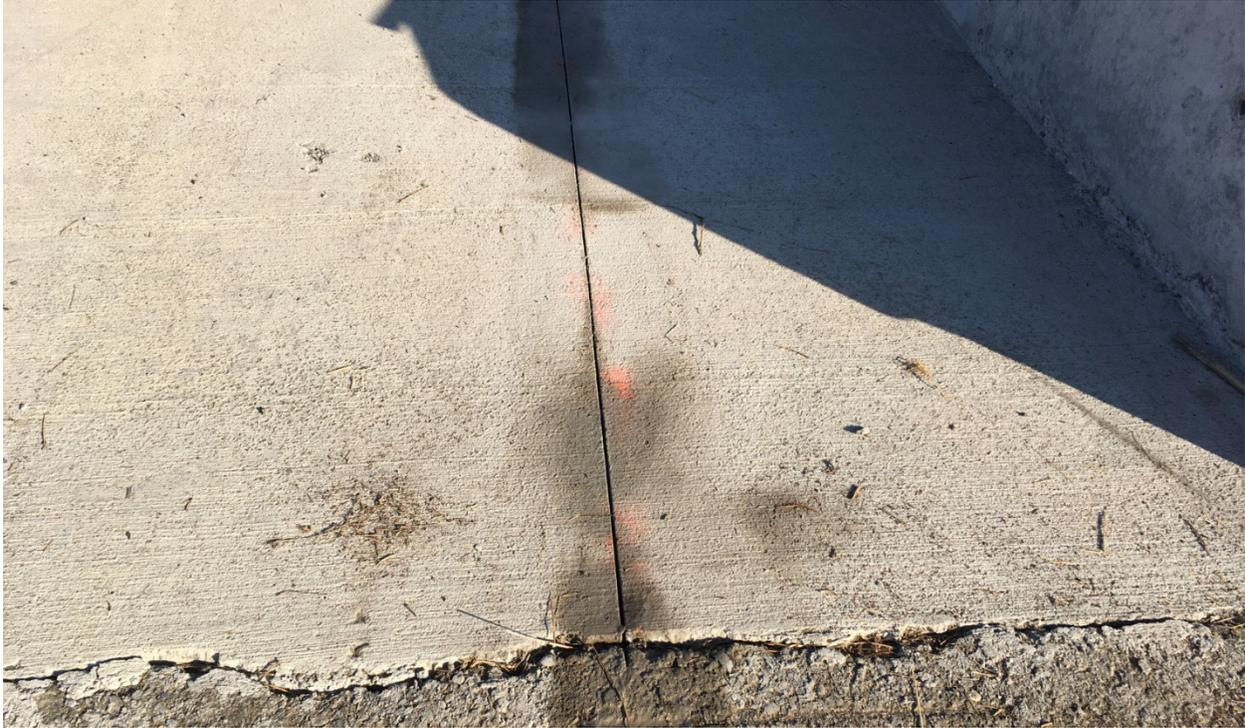
**Figure 2-7 Initial saw-cut line for overhang removal**
