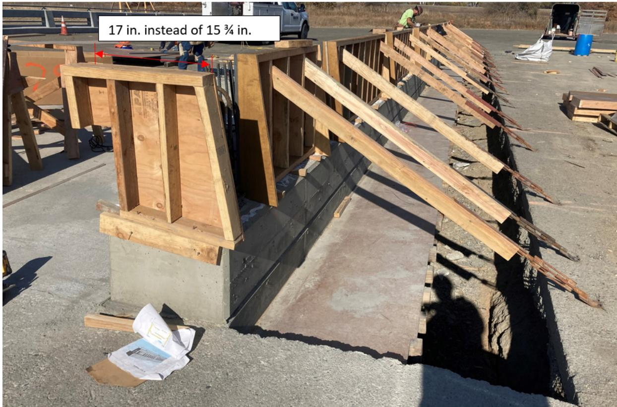
Figure 2-37 Forming of the Back Side and Side of the Structural Post (Post Form increased to 17 in.)
