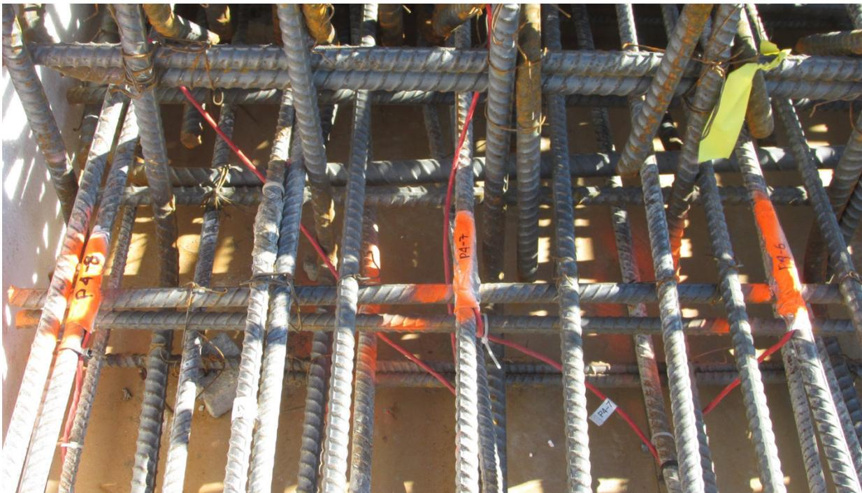
Figure 2-22 Installation of Uniaxial Strain Gauges and Cable at Post 4 Prior to Deck Pour
