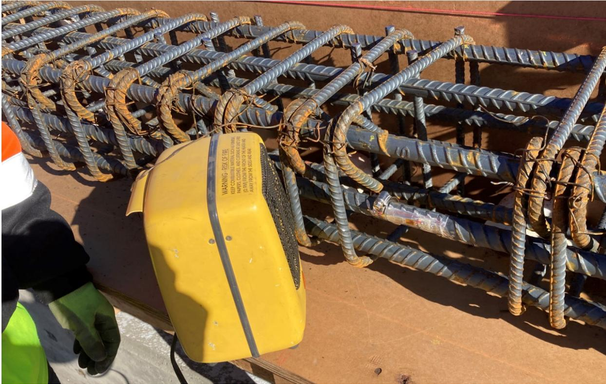
Figure 2-44 Installation of Uniaxial Strain Gauges and Cable Prior to Post and Beam Pour
