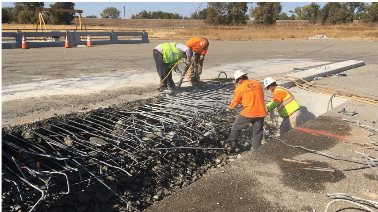
**Figure 2-9 Removal of ST-75 Test Article Overhang at Saw Cut Line with Jackhammers**
