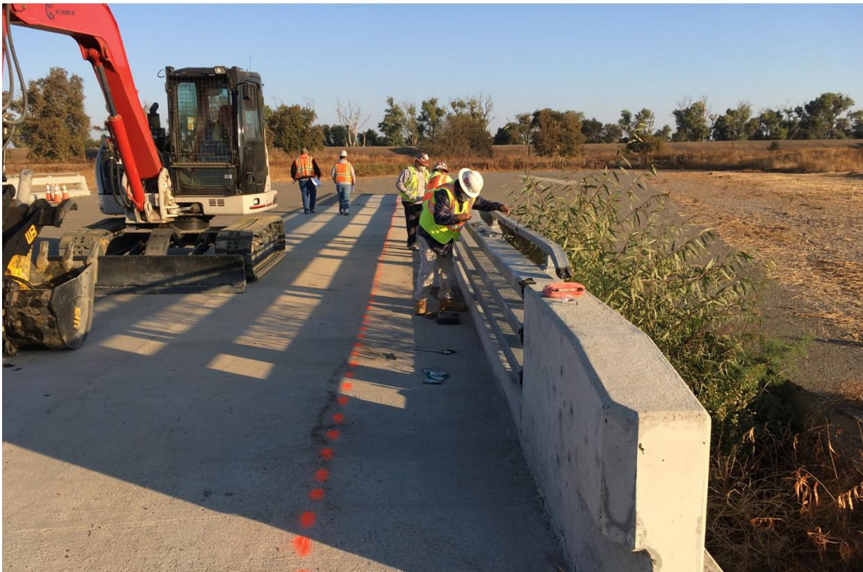
**Figure 2-6 Unbolting of the ST-75 Steel Bridge Rail and Painting of Overhang Saw-Cut Line**
