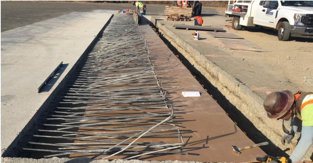
**Figure 2-11 Installation of the Formwork for the Type 86H Overhang and Concrete Curb**
