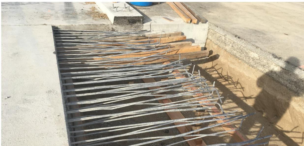
**Figure 2-10 Installation of the Supports for the Formwork for the Overhang Construction**
