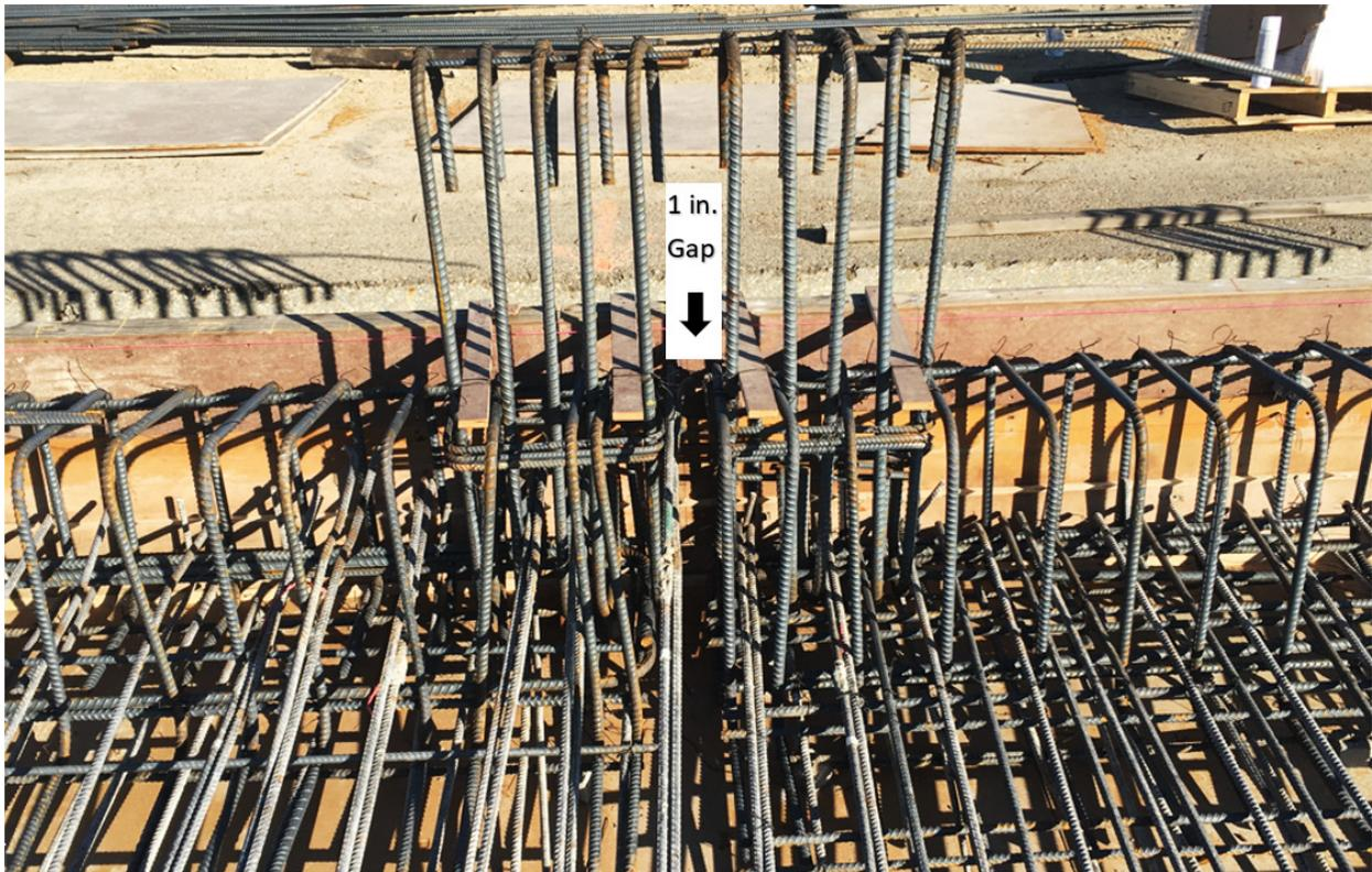
Figure 2-17 Installation of Reinforcement at Posts 4 and 5 with 25 mm (1 in.) Gap
