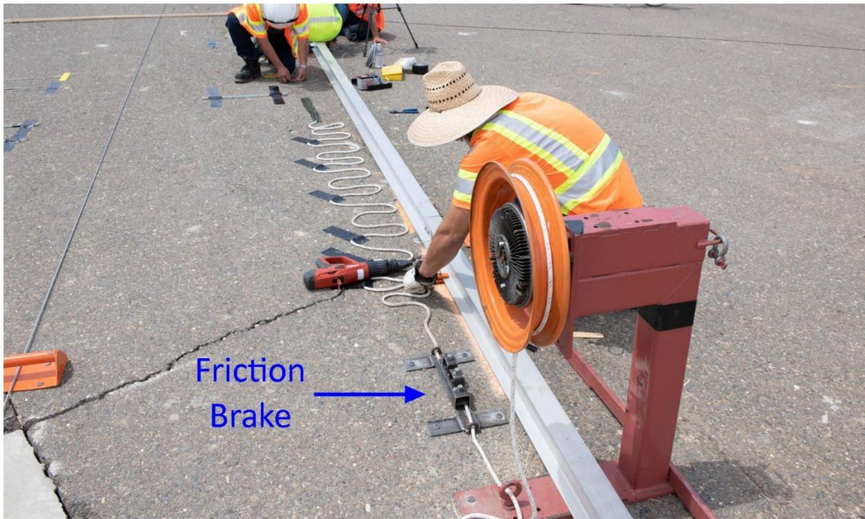
Figure 10-11 Guide Arm Brake System with Friction Brake
