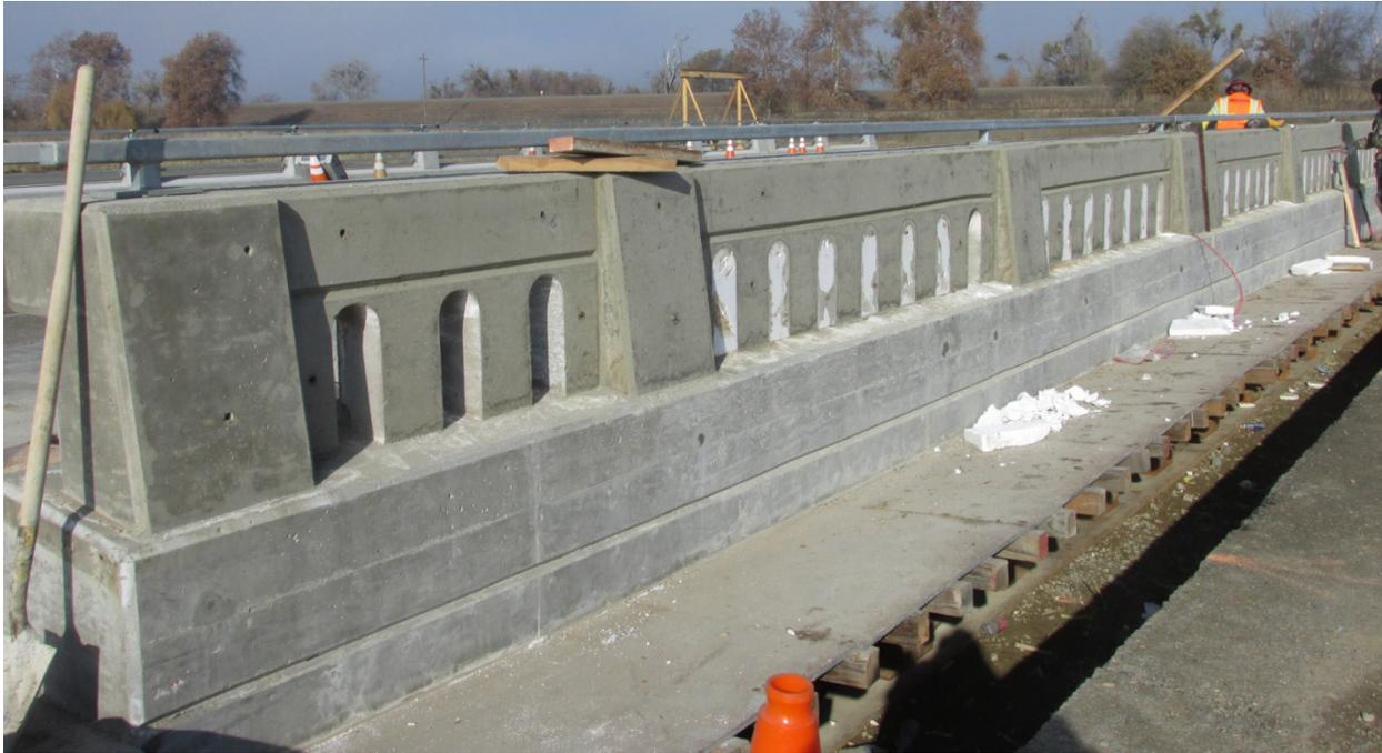
Figure 2-48 Removal of Forms View from the Back
