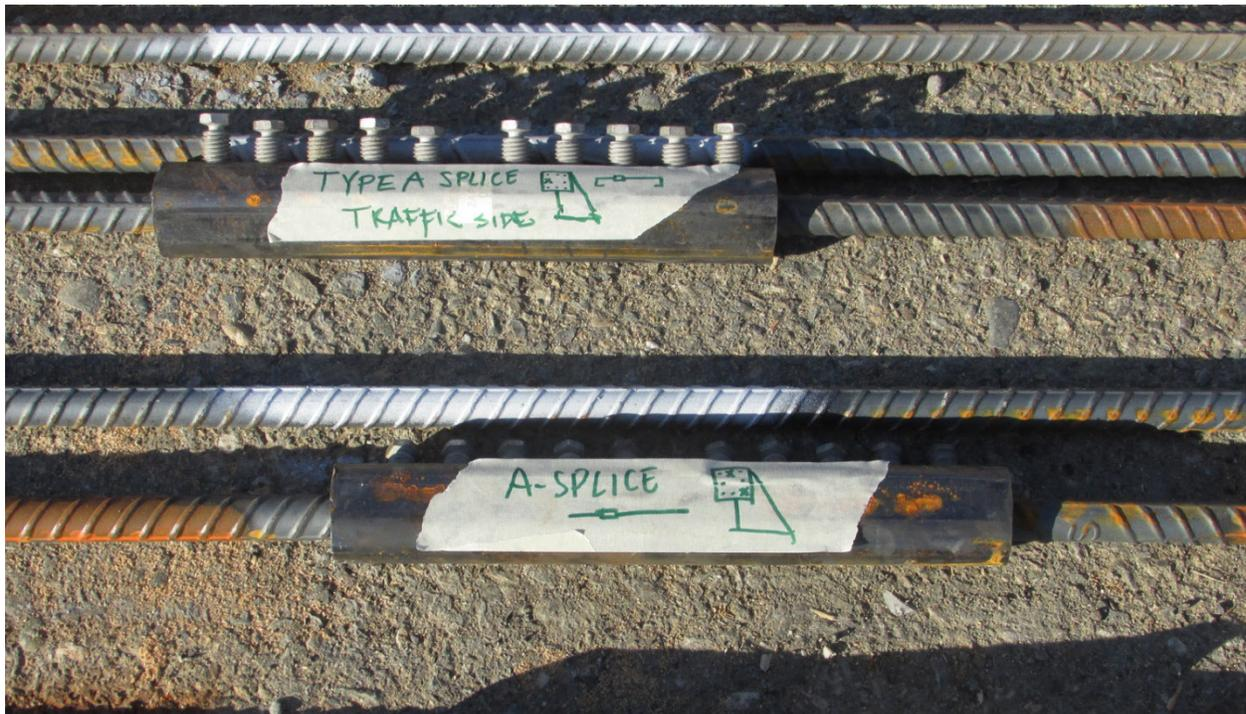
Figure 2-41 Preparation for Splicing of No. 7 Longitudinal Reinforcement
