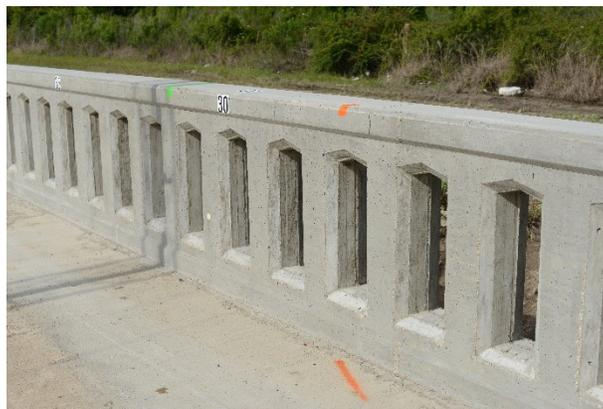
**Figure 1-6 Texas C411 Concrete Baluster Bridge Rail (MASH TL-2)**
