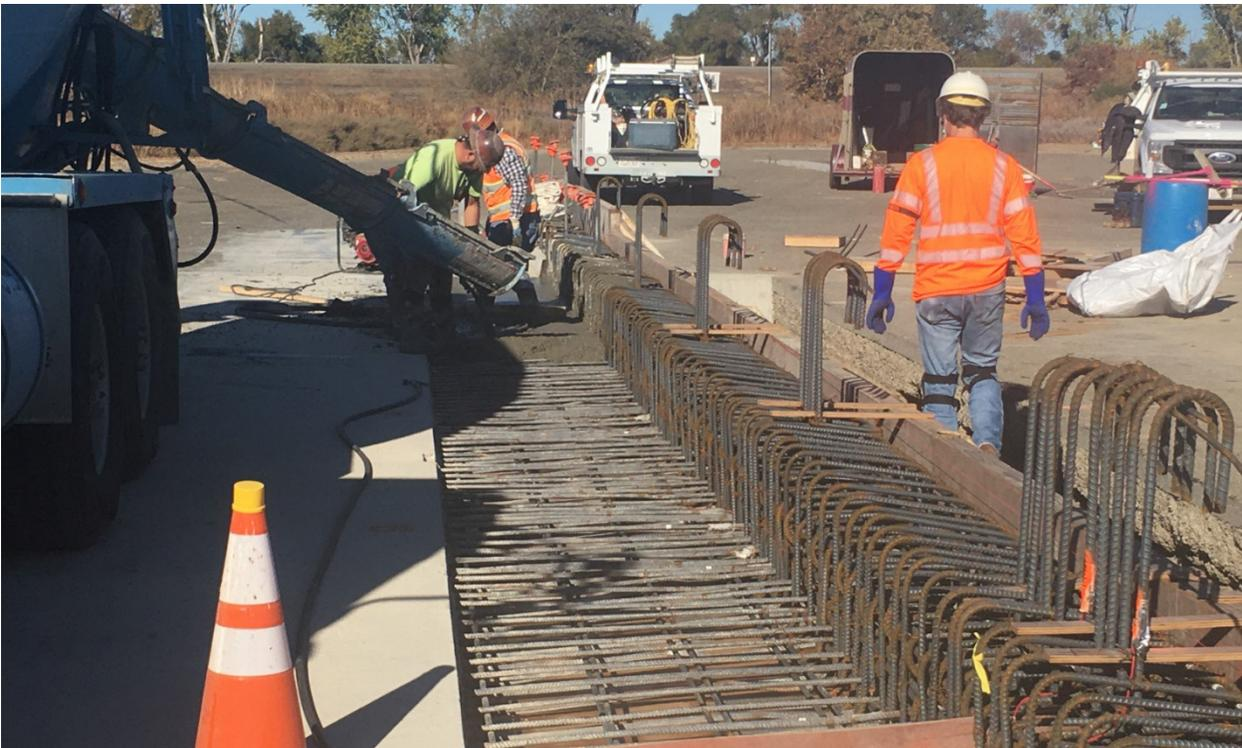
Figure 2-24 Bridge Rail Overhang Concrete Pour
