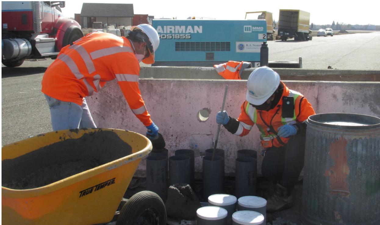
Figure 2-34 Concrete Samples Taken During the Curb Pour by Caltrans Staff
