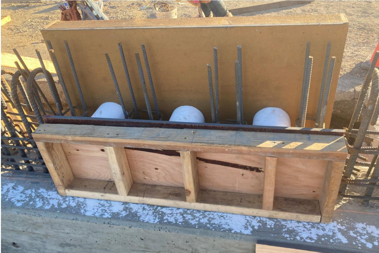
Figure 2-39 Forming of the Baluster Post (placement of the front form)
