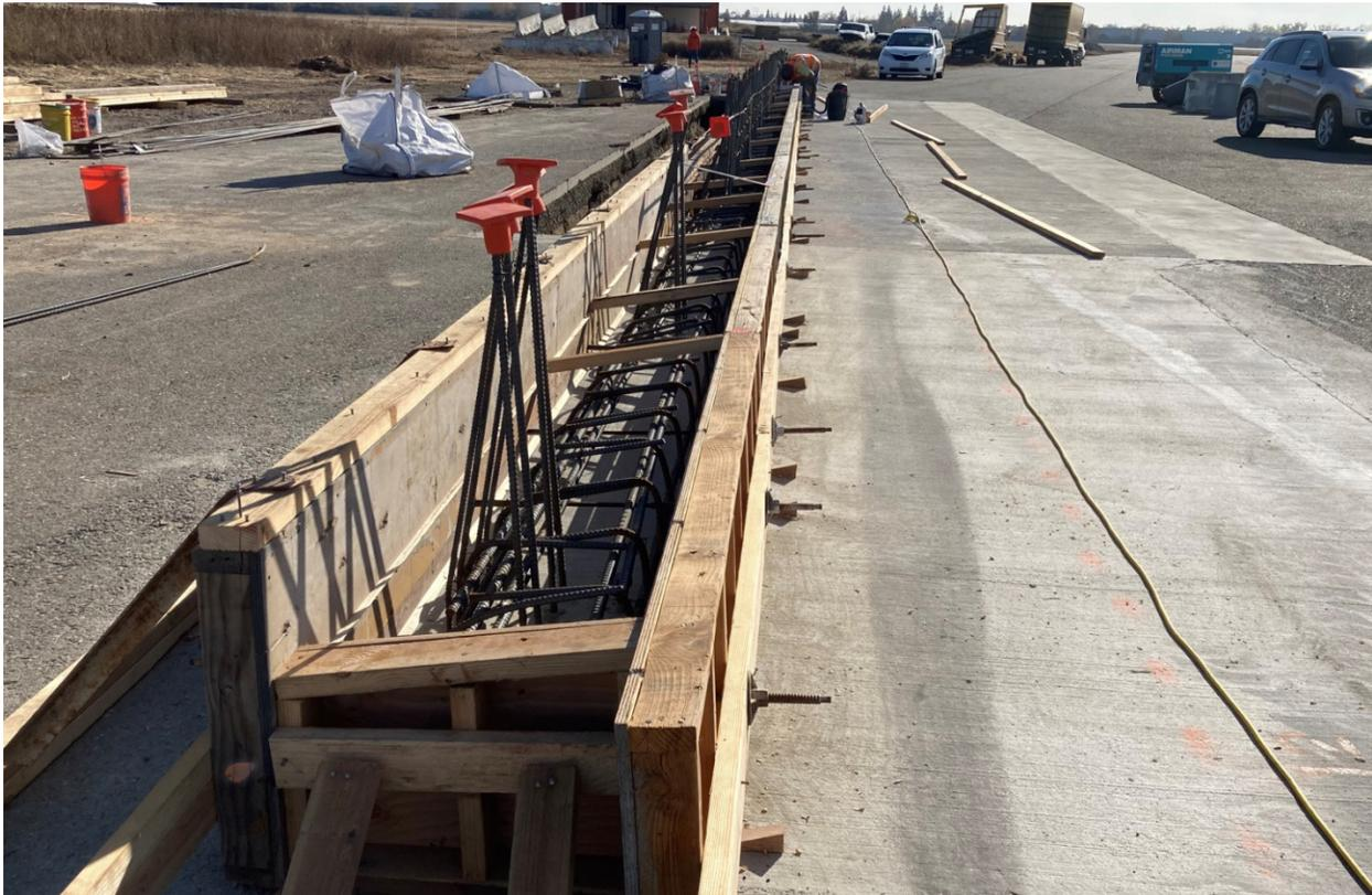
**Figure 2-31 Formwork and Rebar for the Drilled and Bonded Section over the Reaction Slab**
