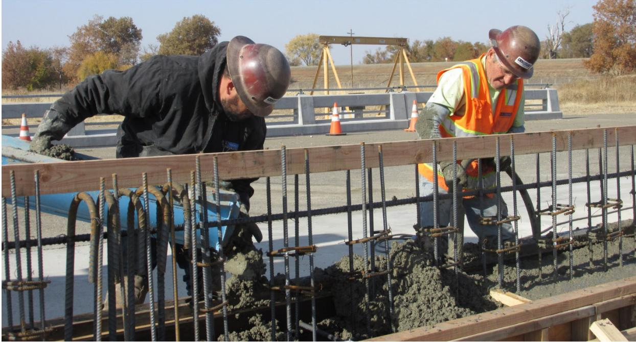
Figure 2-32 Bridge Rail Curb Concrete Pour
