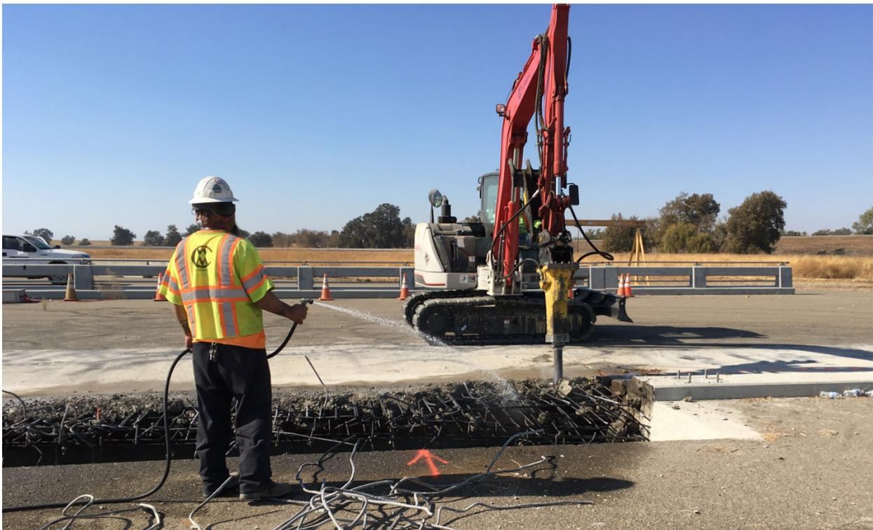
**Figure 2-8 Removal of ST-75 Test Article Overhang with Excavator Hammer Attachment**
