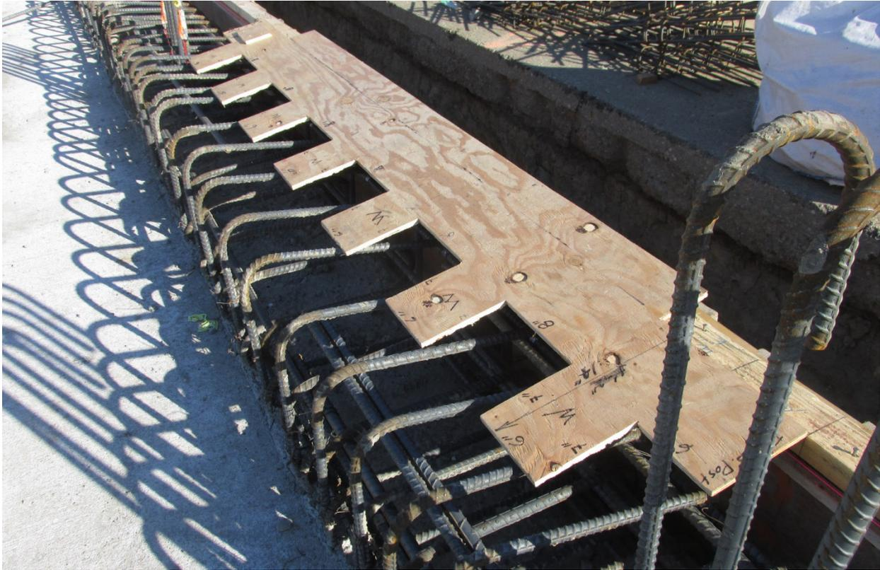
Figure 2-28 Plywood Template Used for Verifying the Placement of Baluster Rail Reinforcement
