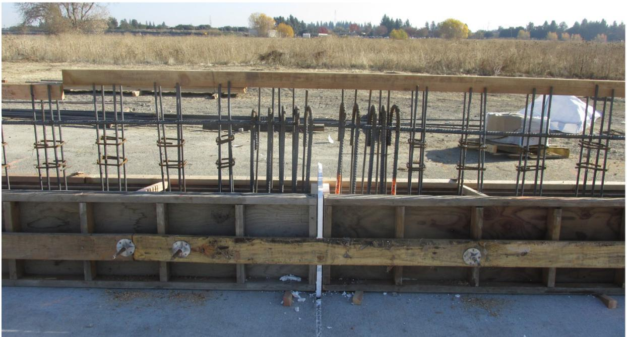
Figure 2-29 Placement of Front Form and Baluster Rail Reinforcement near Posts 4 and 5
