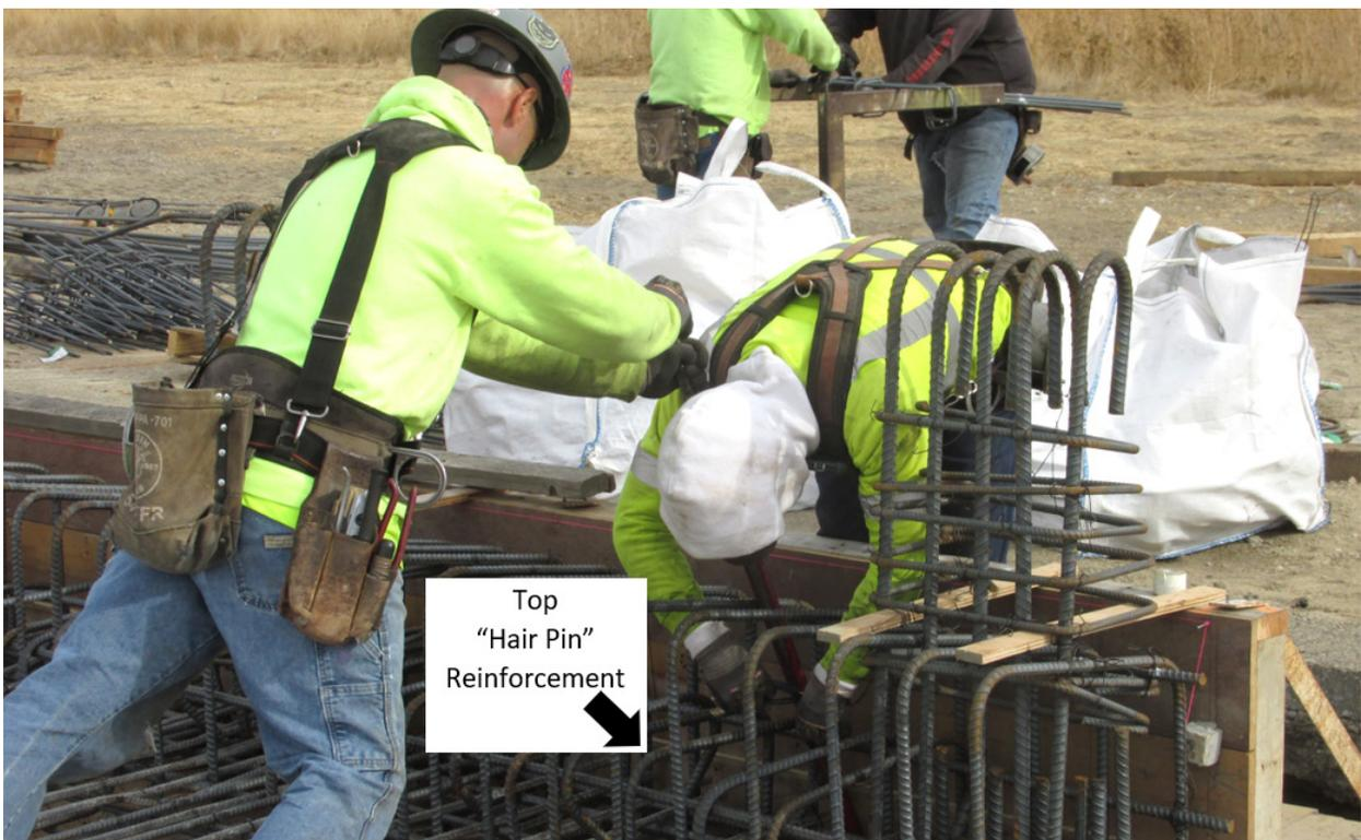
Figure 2-18 Installation of Top #6 Curb "Hair Pin" Reinforcement
