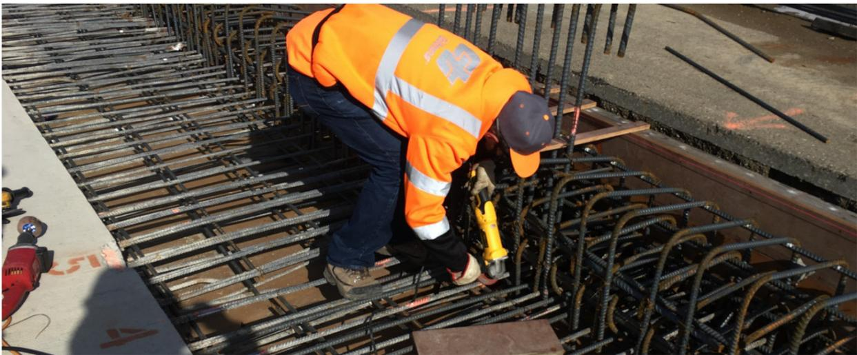
**Figure 2-20 Grinding Surface of Reinforcement in Preparation for Strain Gauges**
