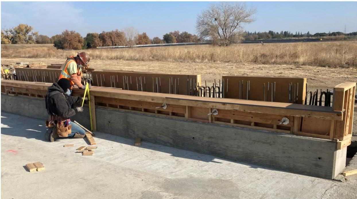
Figure 2-40 Forming of the Underside of the Beam
