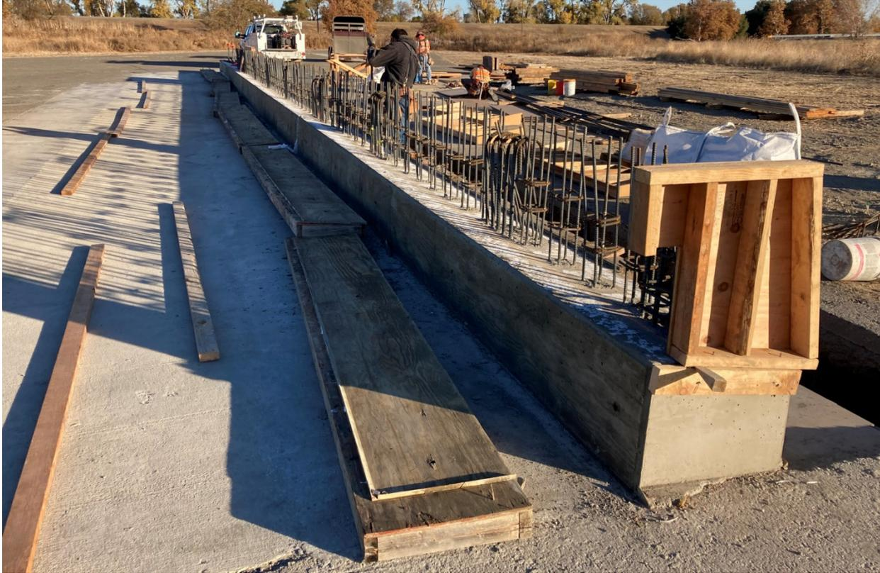
**Figure 2-36 Removal of Concrete Curb Forms**
