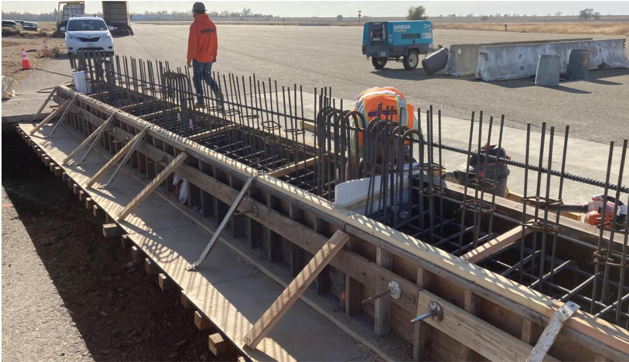
**Figure 2-30 Formwork and Rebar in Place for Bridge Rail Curb Concrete Pour**
