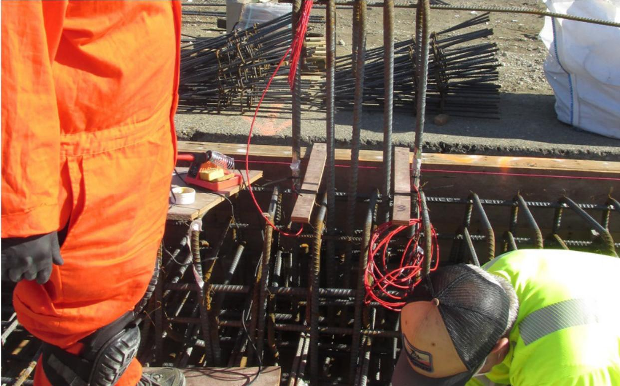
Figure 2-23 Installation of Uniaxial Strain Gauges and Cable at Post 3 Prior to Deck Pour
