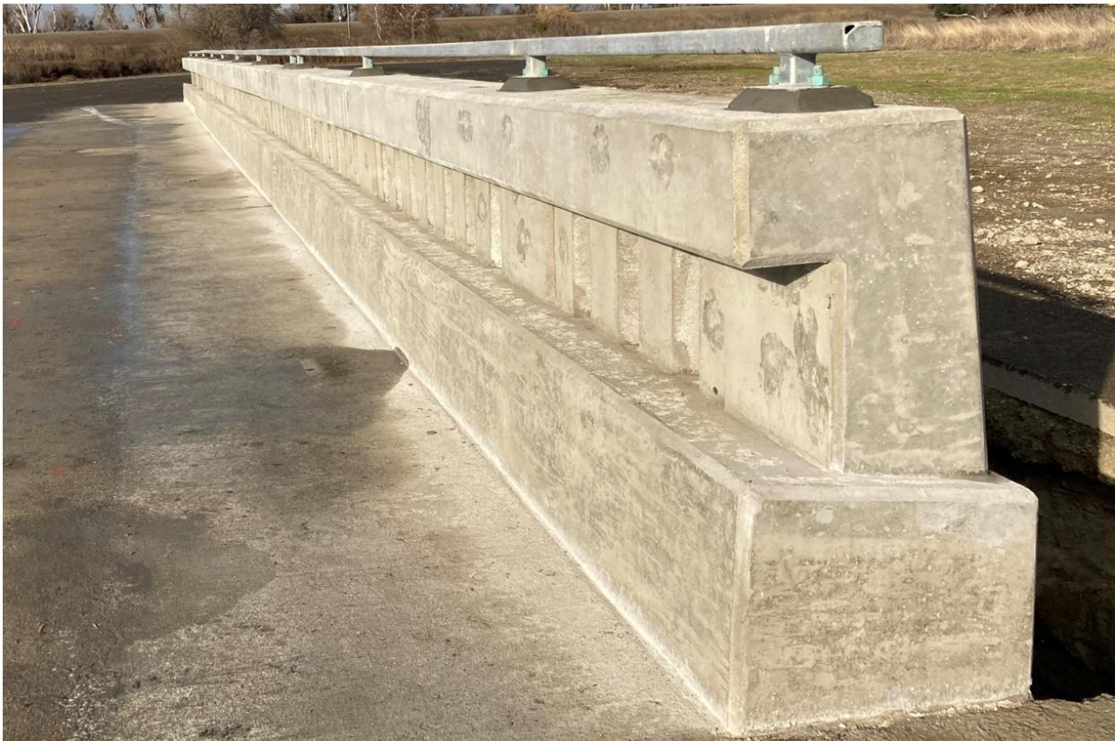
**Figure 2-51 Completed Bridge Rail Type 86H**
