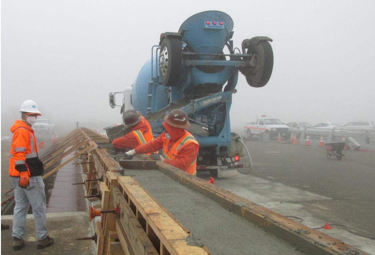
Figure 2-46 Bridge Rail Post and Beam Concrete Pour
