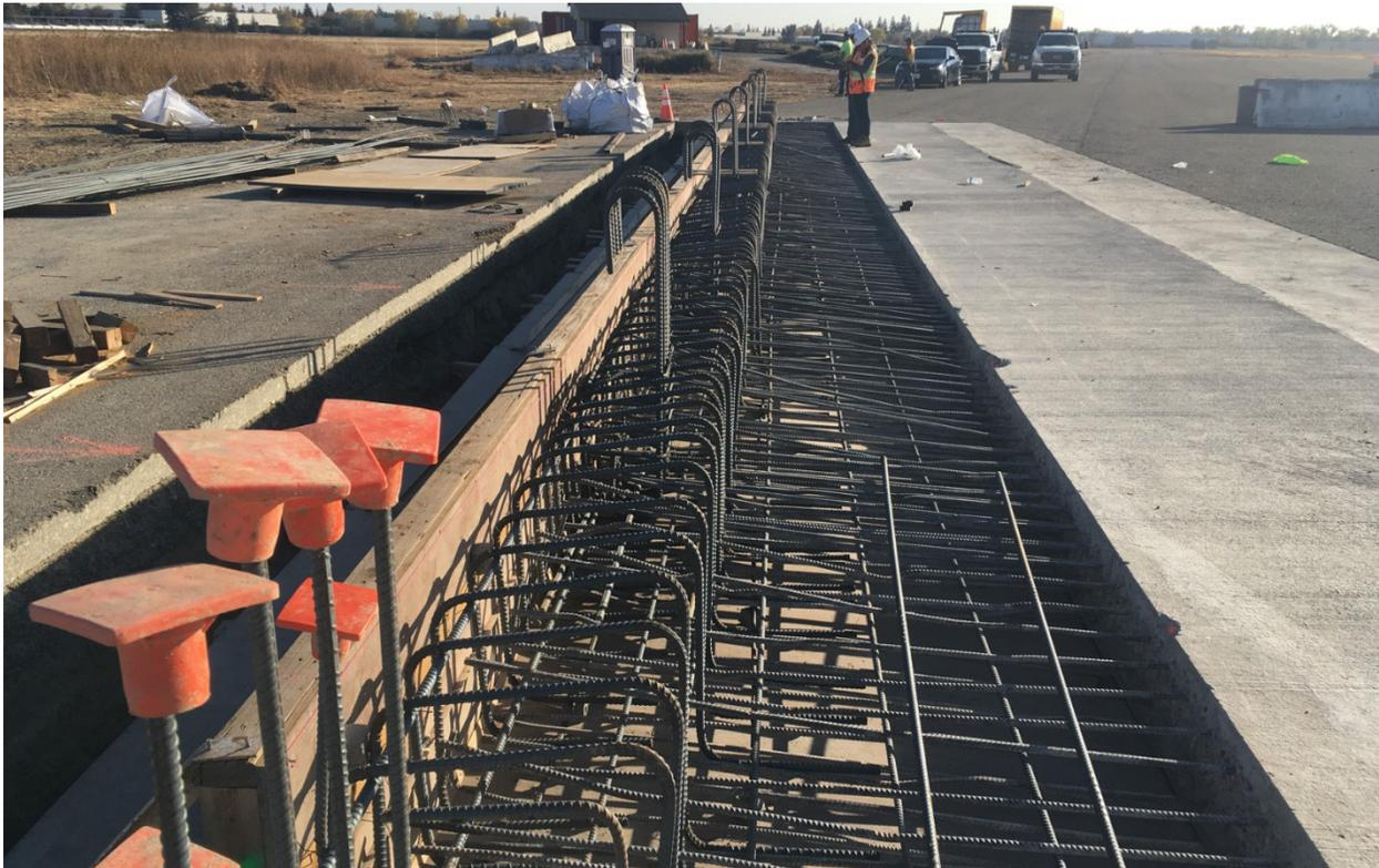
**Figure 2-16 Installation of Longitudinal Overhang, Curb and Post Reinforcement**
