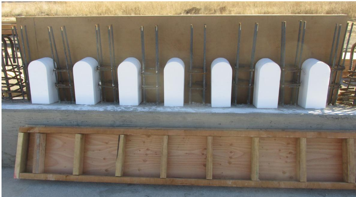
Figure 2-38 Positioning of the Arched Styrofoam Baluster Windows Prior to Installation of Front Form
