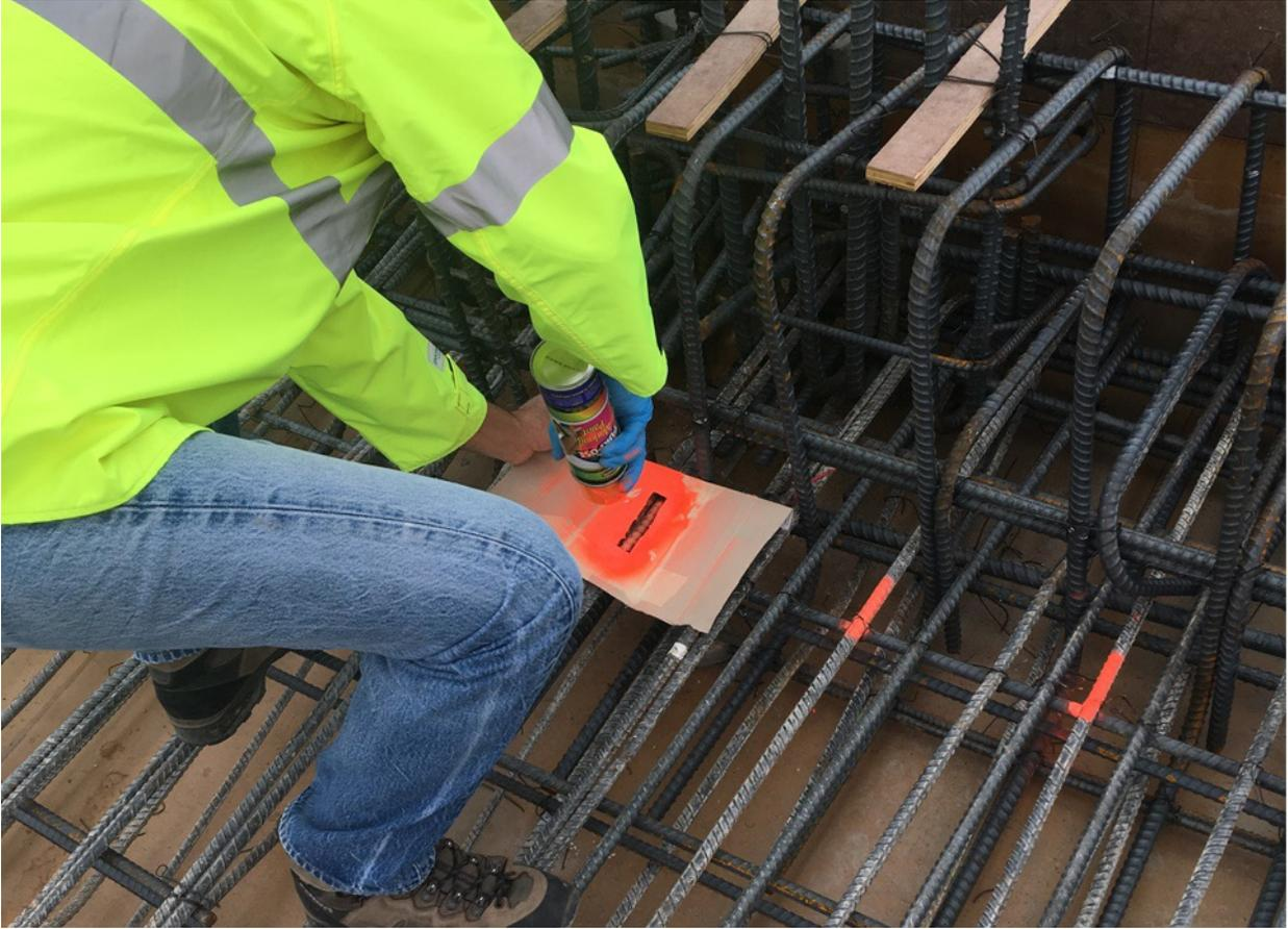
**Figure 2-19 Marking the Strain Gauge Locations on Reinforcement at Structural Post 4**
