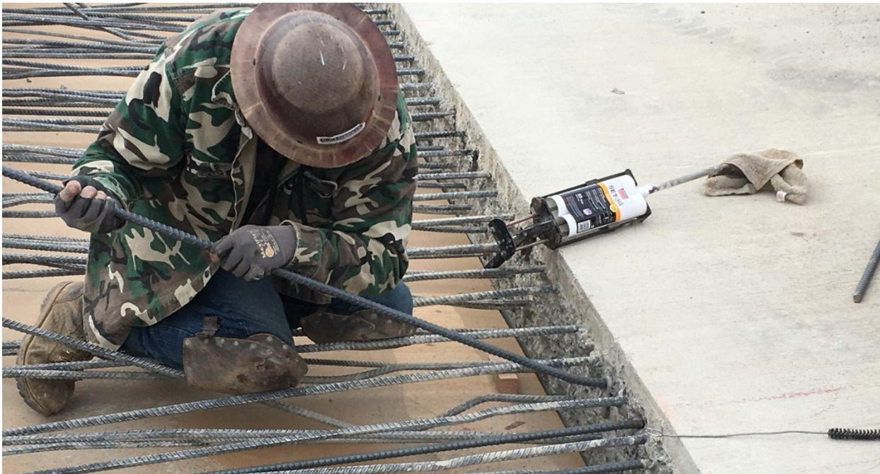
Figure 2-14 Installation of Epoxy and Additional Transverse Reinforcement
