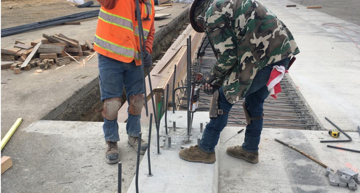
**Figure 2-15 Installation of Epoxy and Vertical Reinforcement on Existing Curb and Reaction Slab**
