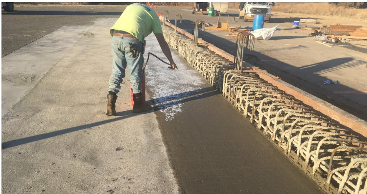
**Figure 2-26 Concrete Finish and Placement of Curing Compound**
