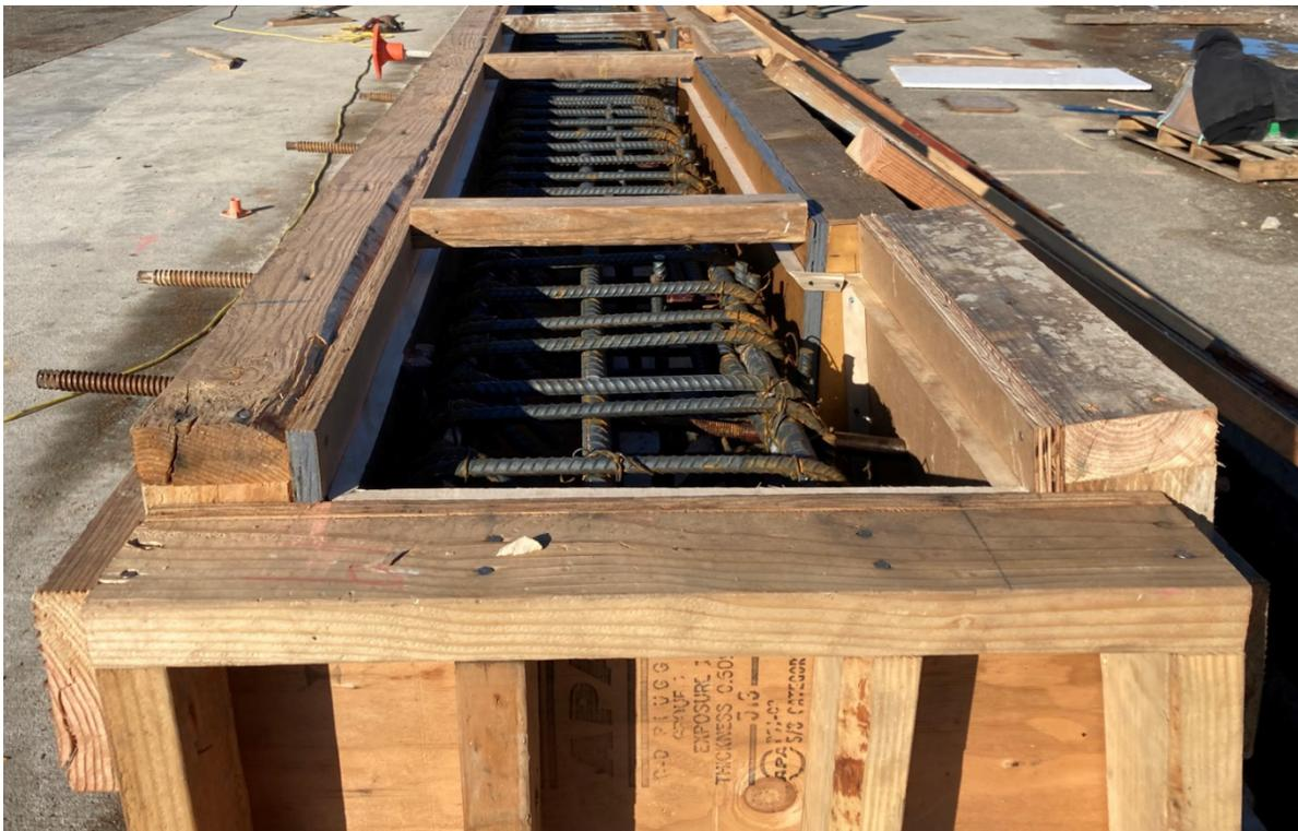
Figure 2-45 Formwork and Rebar in Place for Bridge Rail Post and Beam Concrete Pour
