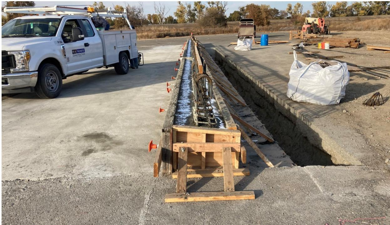
Figure 2-35 Completion of Pour of the Concrete Curb
