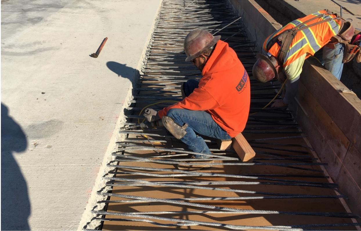
Figure 2-13 Drilling Operation (305 mm (12 in.) depth) for Epoxied Reinforcement Installation
