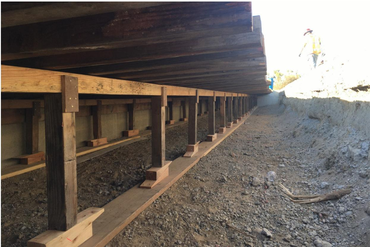
**Figure 2-12 Installation of the Formwork Supports for the Type 86H Overhang and Concrete Curb**
