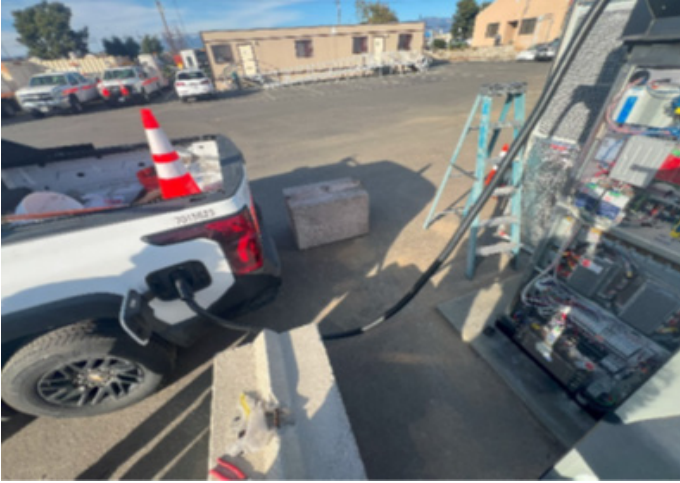
Image 2: Testing FreeWire Boost Charger 200 during final commissioning process.
