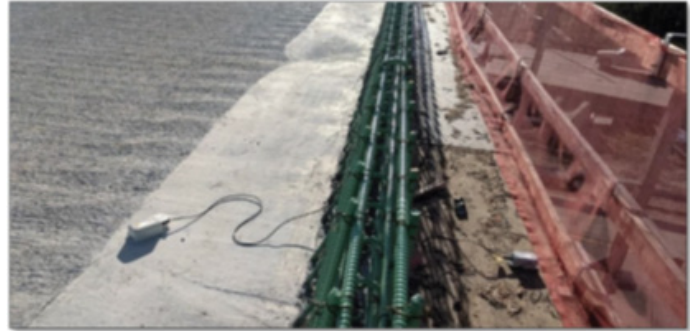
Image 1: Hardware of REBEL concrete strength monitoring system.
