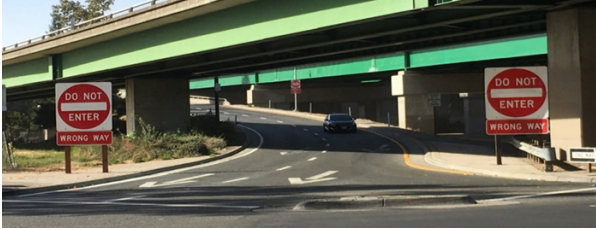
Image 7: Exit ramp with enlarged DO NOT ENTER / WRONG WAY signs
