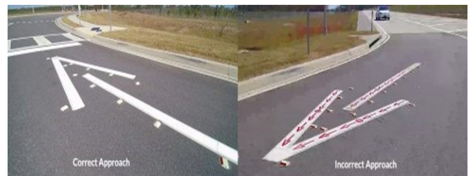
Image 7: Bidirectional pavement markings
