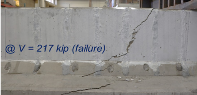
Image 3: Failure of strengthened specimens (Phase I): (a) NSM.
