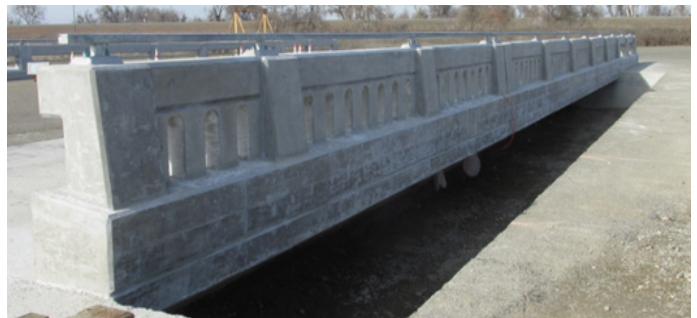
Image 2: Backside View of The Type 86H Concrete Barrier Rail
