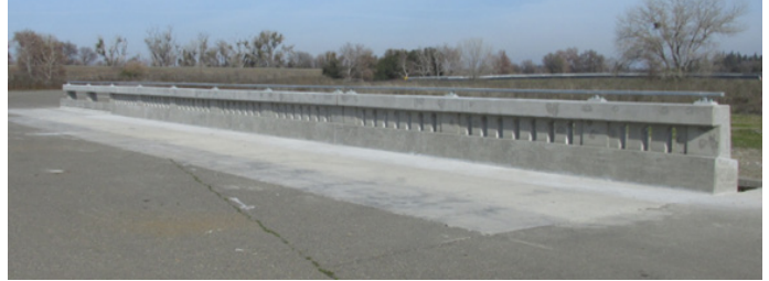
Image 1: Front View of The Type 86H Concrete Barrier Rail
