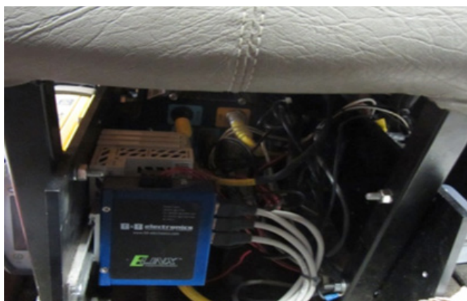
FIGURE 4: DAS computer installed underneath passenger seat
