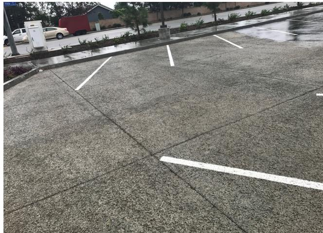
Figure 5: Fully permeable concrete pavement
