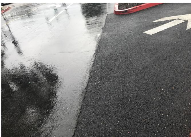
Figure 4: Comparison of conventional (left) and fully permeable asphalt pavement (right).
