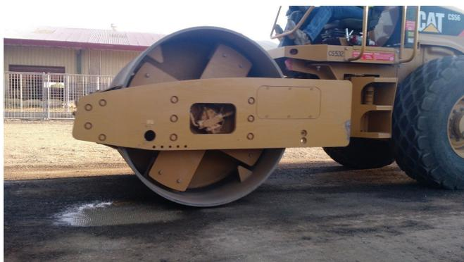
Image 2: Roller microcracking the newly cemented base at 24 hours.
