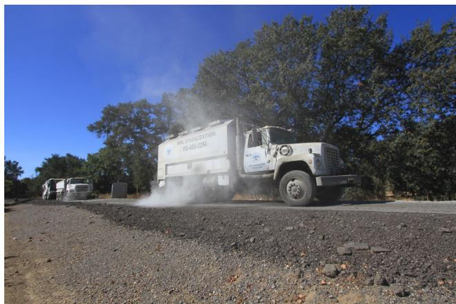
Image 1: Cement placement prior to being mixed into the asphalt and base
