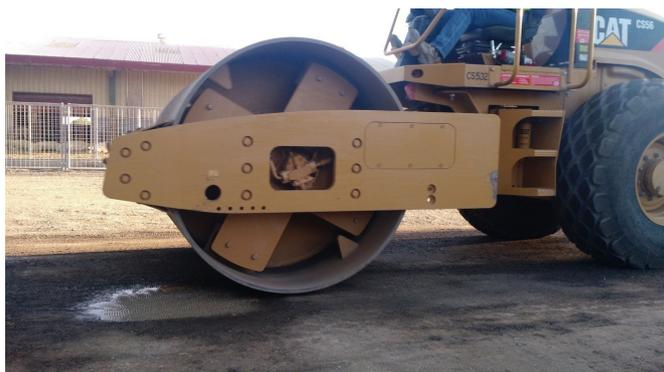
Image 2: Roller microcracking the newly cemented base at 24 hours.
