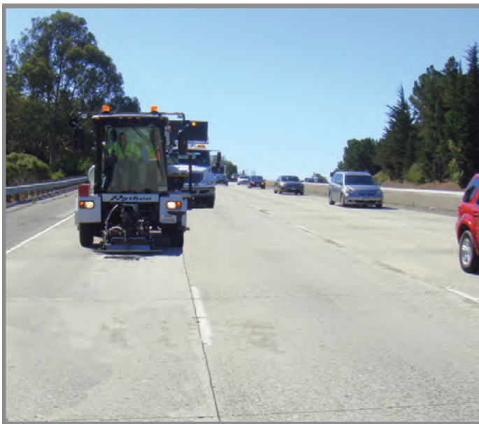
Python automated hot asphalt patching
