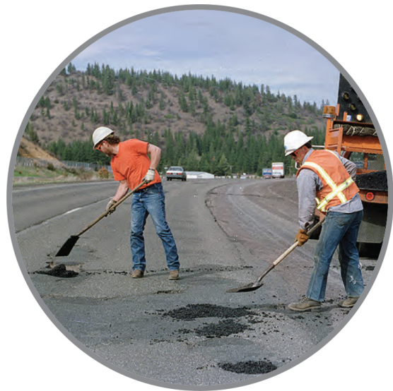
Manual pothole patching
