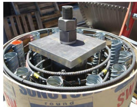
Figure 1: Pipe pin in pedestal
