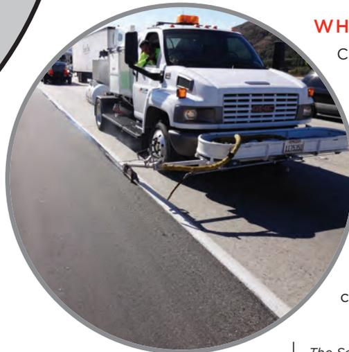
*The Sealzall longitudinal sealing operation produces a uniform and smooth seal, shown here on Interstate 15 in Escondido.*
