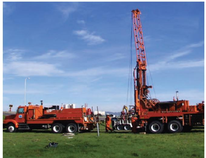
Figure 2: Drilling a downhole array at the Napa River bridge
