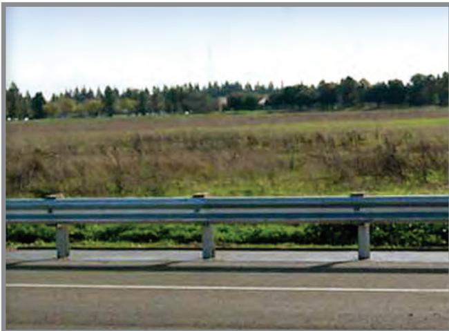
*CRMCrete weed control barrier, made from readily available recycled products, blocks weed growth under guardrails, reducing recurring maintenance activities, such as herbicide application, pruning, and mowing.*
