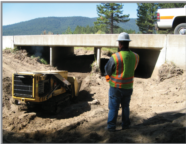
Operator controlling loader. Fletcher Creek, Highway 89, District 3
