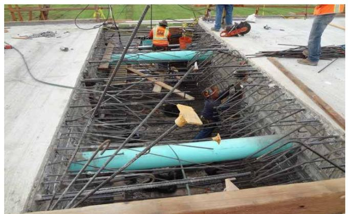
Image 2: Construction of an in-span hinge (Del Paso Park Overhead, Sacramento)
