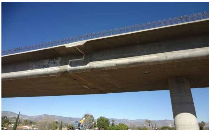
Image 3: In-span hinge of CIP/PS box girder bridge (N170-N5 Connector, Los Angeles)
