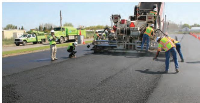
Figure 1: Rubberized warm mix asphalt paving at the Pavement Research Center
