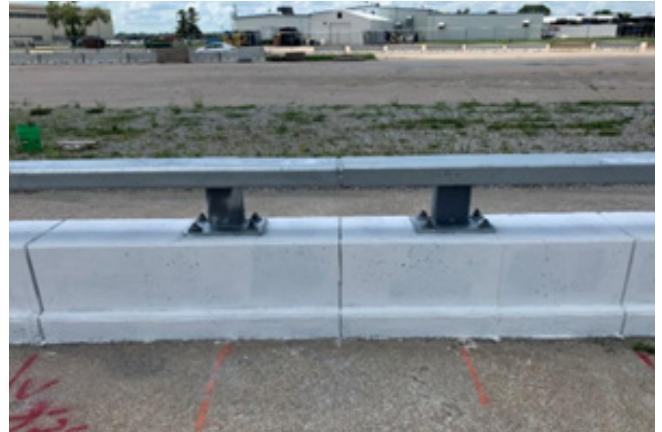
Image 2: Close up View of Barrier at a Rail Splice
