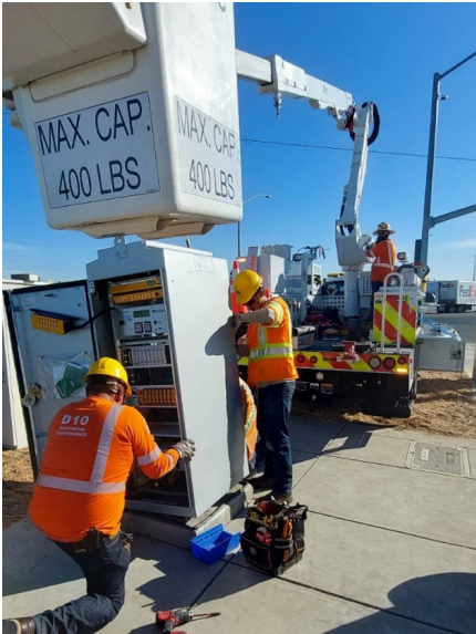
Image 1: Installation of Swarco ATC Cabinet on French Camp Rd.
