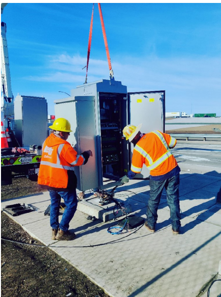
Image 1: Safetran ATC Cabinet Installation
