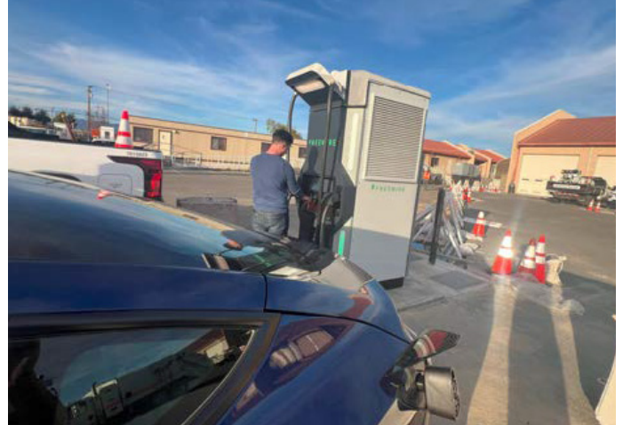
Image 2: Testing FreeWire Boost Charger 200 during final commissioning process.
