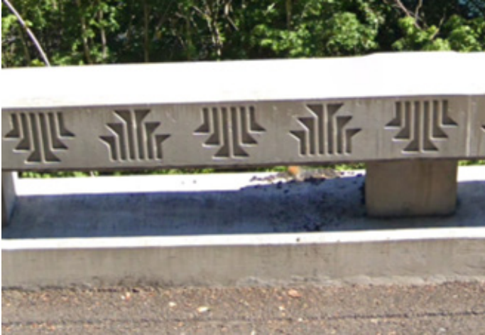
Image 2: Example of textured post-and-beam bridge rail.
