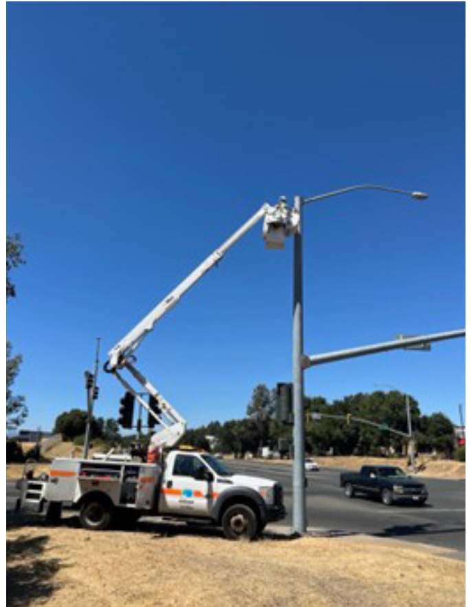
Image 2: Field staff installing camera and LiDAR equipment at Dam Rd & CA 53, Clearlake, CA.
