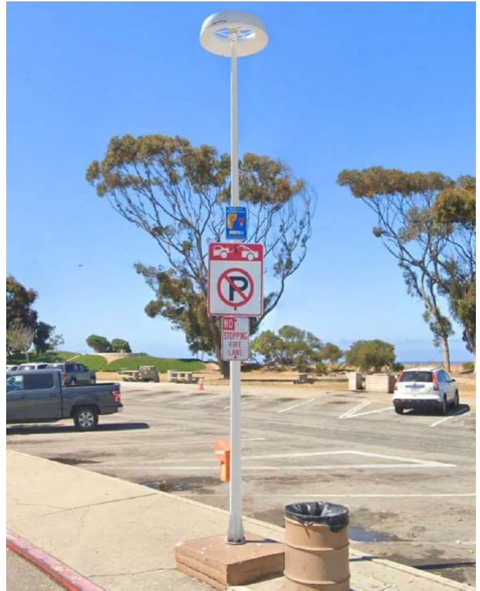
Image 1: An example Omniflow OMNILED unit mounted to a pole that was installed in District 11.
