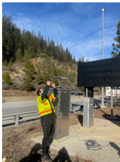
Image 1: Image shows researcher determining best orientation for satellite dish while testing equipment at a field site – Image Source - Caltrans
