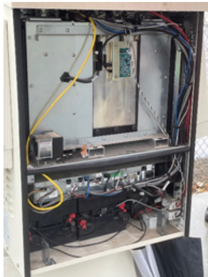
Image 3: Hydrogen Fuel Cell – Image Source - Caltrans
