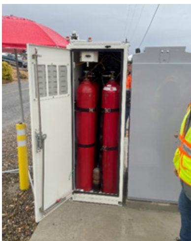
Image 2: Hydrogen Fuel Cylinder cabinet – image Source – Caltrans
