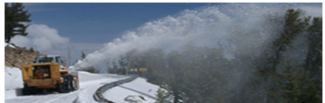
Image 1: Rotary blower removing snow from roadway
