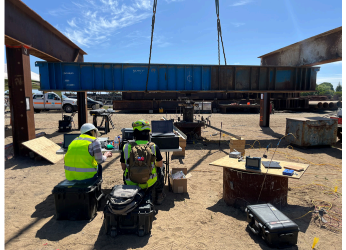
Image 2: Pile Load Testing
