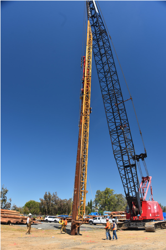
Image 1: Pile Installation
